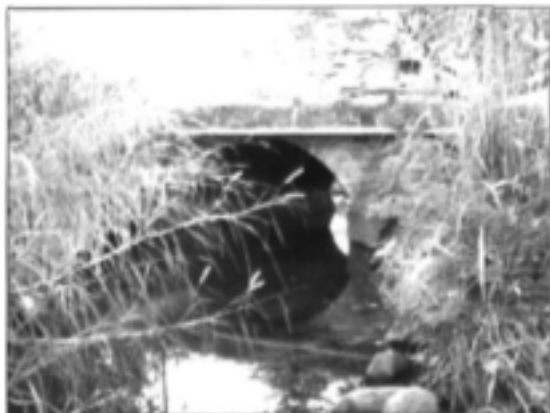
Plate 18.1. Galway Road bridge at top of Reach 18 (looking upstream). This bridge had to be stabilised following the 2002 floods.
