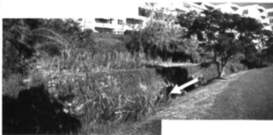
Plate 5.4. Lower end of the reach, showing the vegetated gabion stabilisation on the right bank of the river. Channel and flow direction shown with an arrow.
