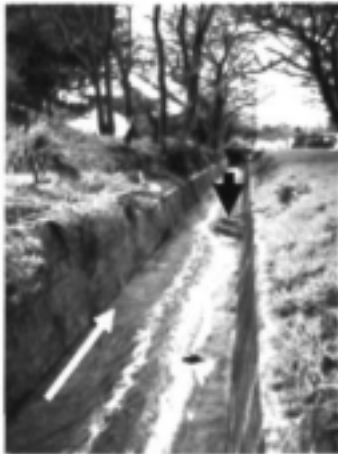
Plate 1.1 The river first daylights into this canalised section. There is a manhole halfway along the canal. Flow direction shown.
