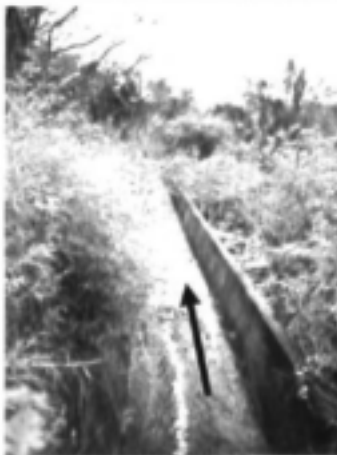
Plate 2.2 Canalised section of the river, downstream of Neale Road. Direction of flow shown
