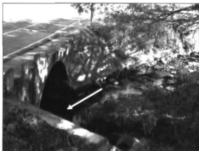
Plate 17.3 Galway Road bridge. Note angle of bridge relative to channel.
