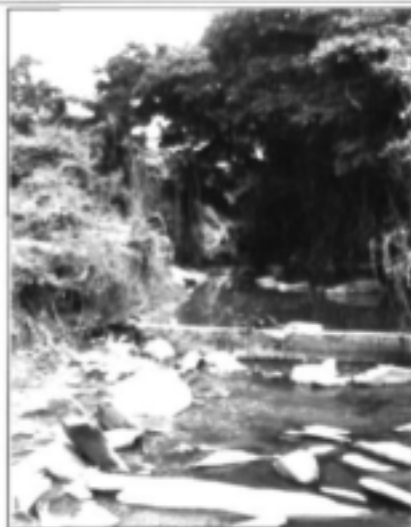
Plate 25.1 Looking upstream towards weir
