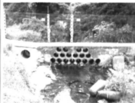
Plate 8.1 Culvert bridge at the upper end of Reach 8
