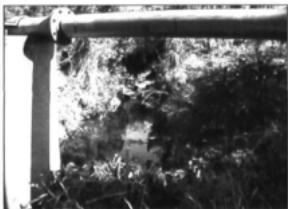
Plate 24.1 Upstream of the pipebridge over the channel
