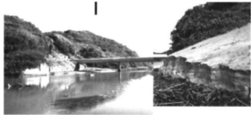
Plate 30.1 The mouth of the Ihlanza looking from the left bank. Note the concrete bollards used to stabilise the dune (one large section of stabilisation is washed out).
