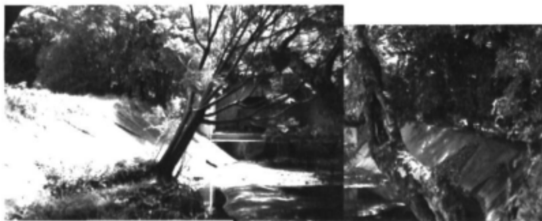
Plate 10.1 Stilling well at top of Reach 10, receiving flows from the box culvert which runs beneath North East Expressway and Old Transkei Road
