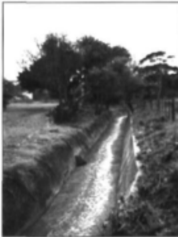
Plate 13.1 Concrete canal in Reach 13.
