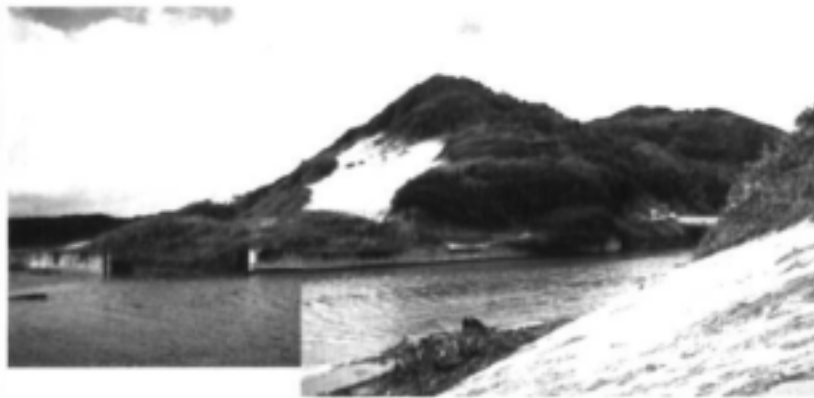
Plate 30.1 The mouth of the Ihlanza looking from the left bank. Note the concrete bollards used to stabilise the dune (one large section of stabilisation is washed out).
