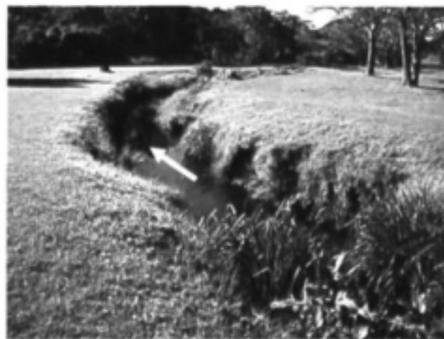
Plate 6.1 U-shaped earth channel in Reach 6.
