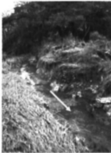
Plate 11.1 Lower Reach 11, soon after August 2002 floods.
