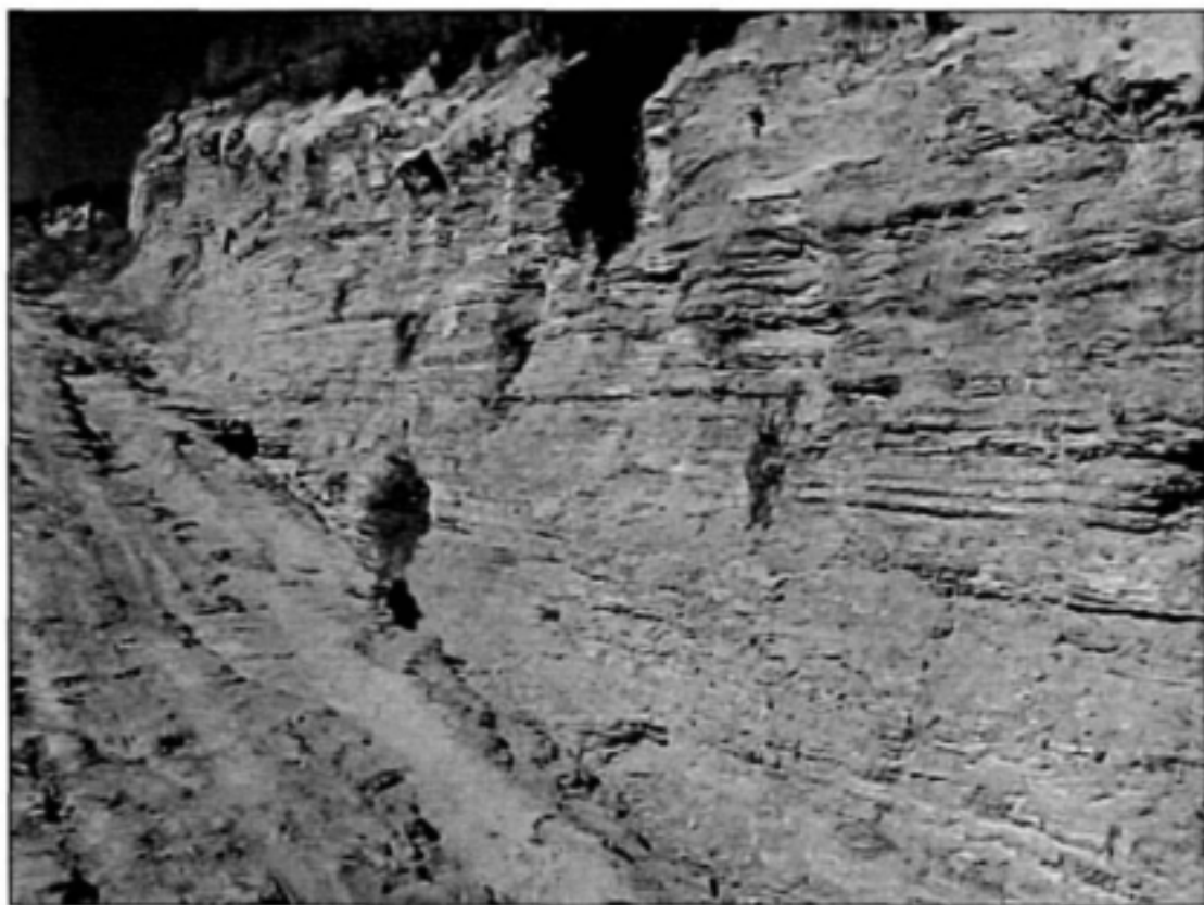
Figure 2.1.1(a): Stratification visible within a wall cross-section of an FRD.
