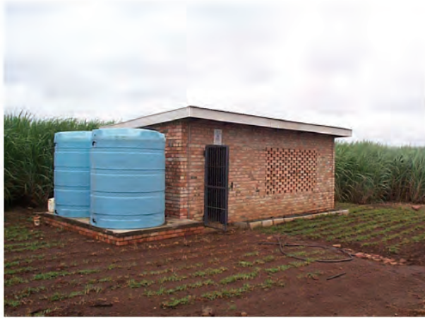
Photo 1: Cluster house external view with fertiliser tanks
