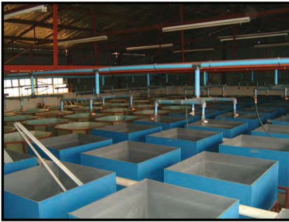
The indoor facilities at Turfloop Hatchery are in a good state of repair and well suited to large-scale fingerling production.
