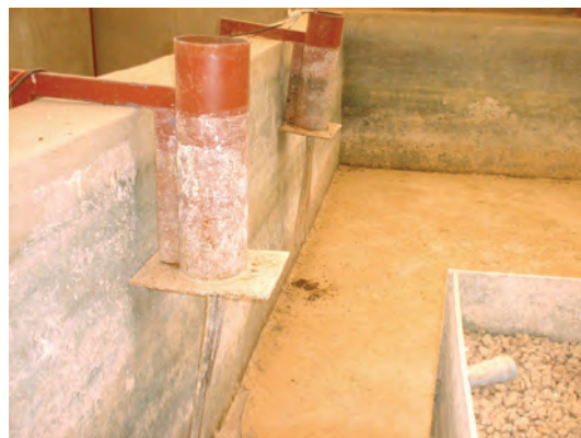
Figure 5. Insufficient gravel remains in the primary filter chambers to be effective, but should be better situated in the secondary chambers, leaving the primary chambers as settling tanks. The secondary chambers currently house numerous high wattage geyser-type heating elements which should be removed, and replaced with a heat-pump for additional heating if required.
