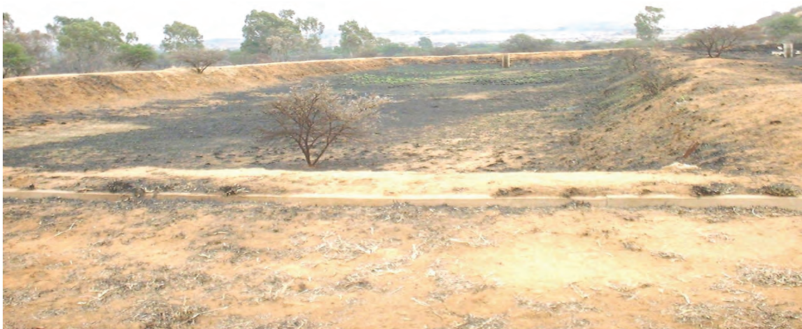
Figure 9. Large rough earthen ponds with no predator-proofing. Each pond is fitted with a monk-type drain. Such ponds would need bird netting, platanna-proof walling and fencing to be of much value.
