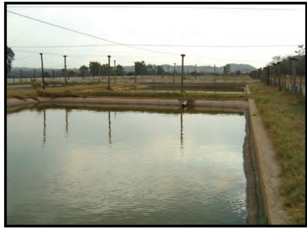
The outdoor ponds at Turfloop are in a good state of repair. Note the support system for bird netting is still intact.
