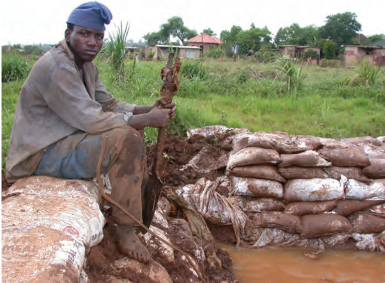
Figure 10. A labourer at a rural farm in Limpopo taking a rest from building the walls to a pond
