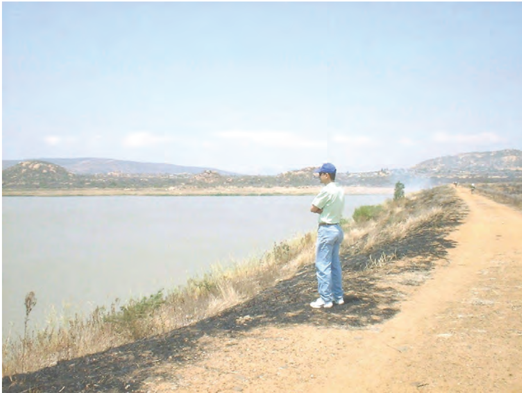
Figure 1. Turfloop Dam, October 2006. The dam is being burnt by nearby community farmers for cattle grazing, and is badly eroded on its flanks as a result.
