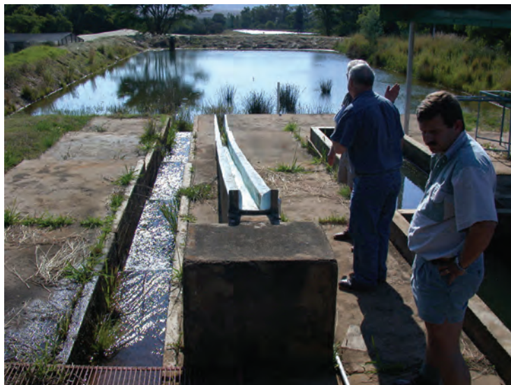
Figure 50. There is considerable infrastructure at Lydenburg Trout Hatchery
