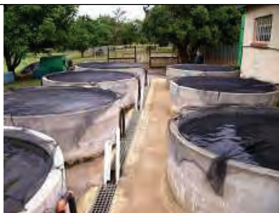
Figure 2: The original 7 concrete tanks constructed at the Research Station in the 1980s
