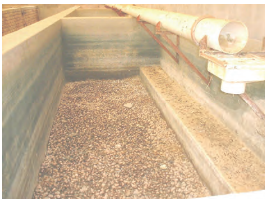
Figure 5. Insufficient gravel remains in the primary filter chambers to be effective, but should be better situated in the secondary chambers, leaving the primary chambers as settling tanks. The secondary chambers currently house numerous high wattage geyser-type heating elements which should be removed, and replaced with a heat-pump for additional heating if required.
