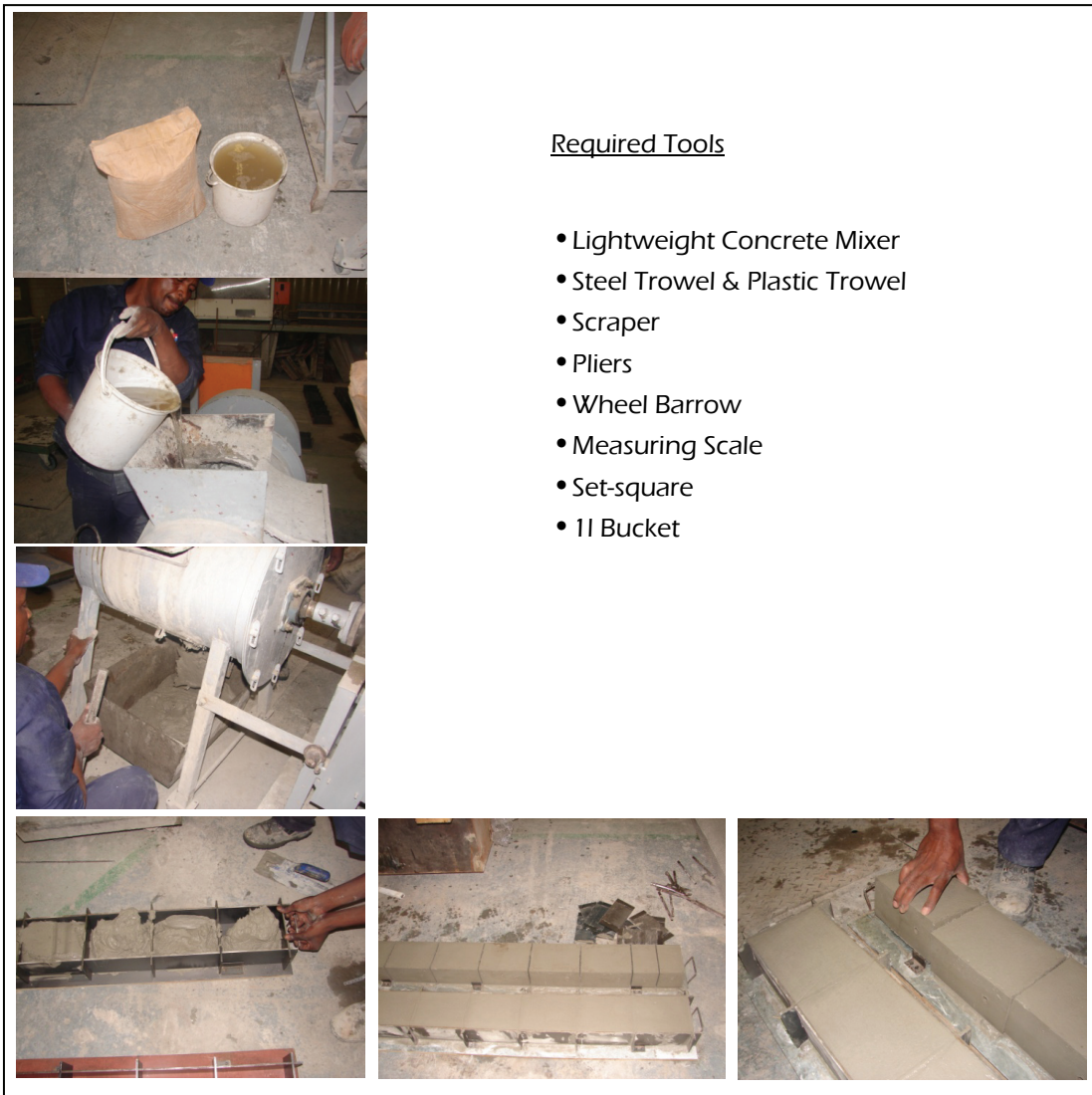
Figure 31: Casting foamed concrete blocks
