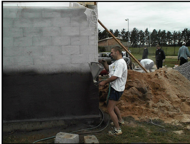
Figure 23: Spraying of surface
