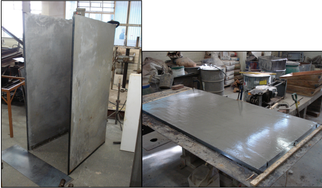
Figure 14: Casting of high strength panels
