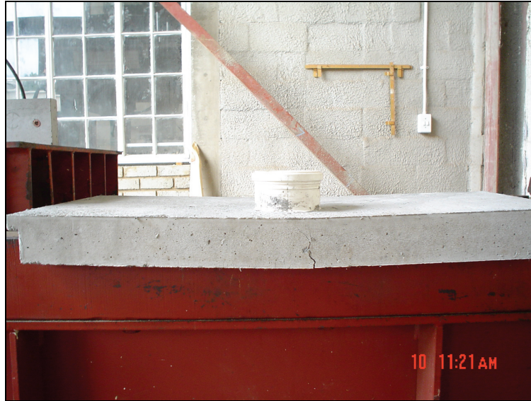
Figure 36: Panel with opening after testing
