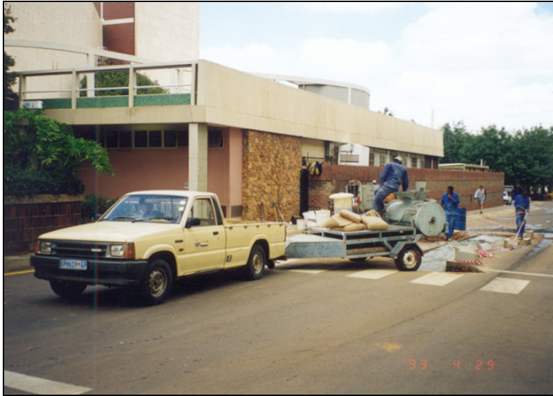
Figure 21: Equipment required for making foamed concrete blocks
