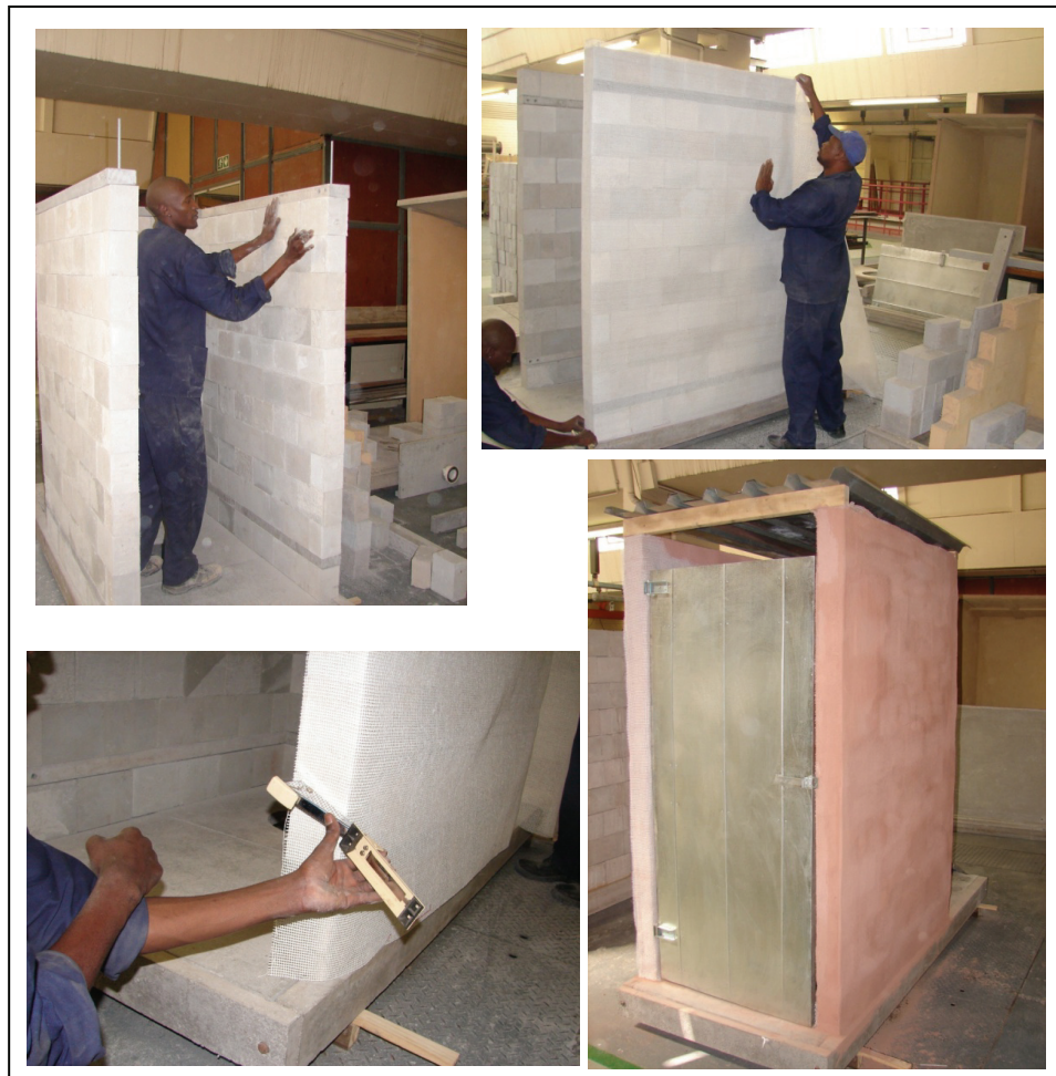
Figure 32: Stacking and wrapping of block structure
