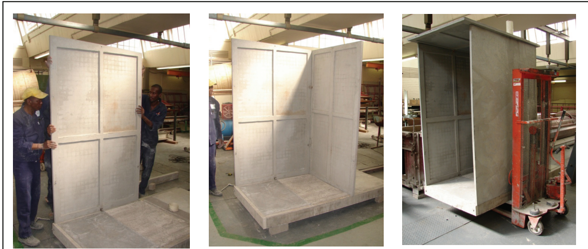
Figure 29: Photos of panel assembly
