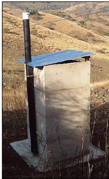
Figure 3: Pre-cast C-sections (SAICE, 2007).
