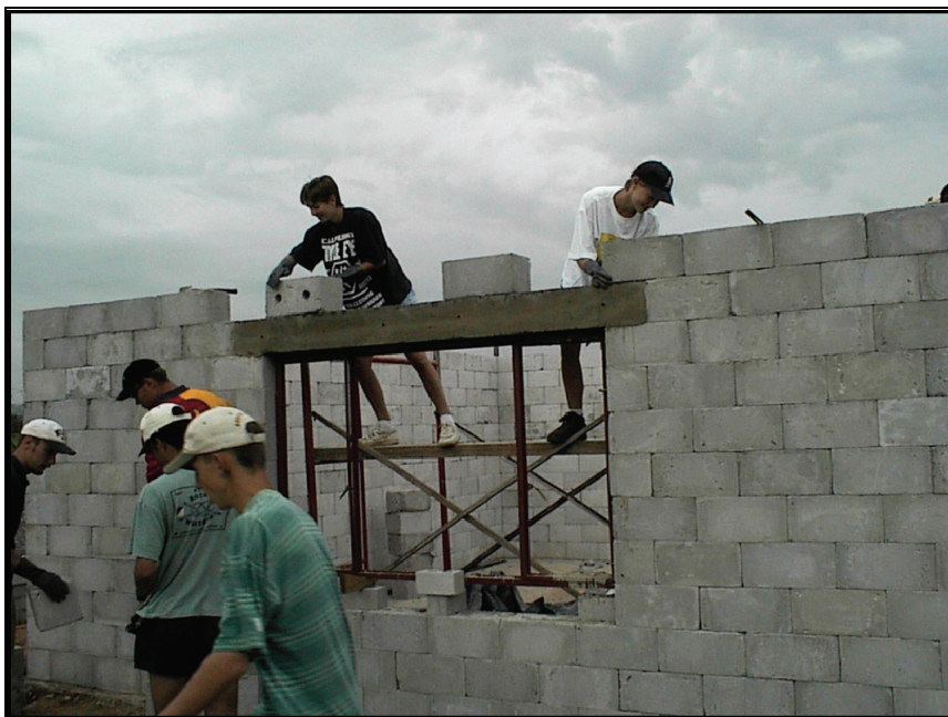
Figure 22: Dry stacking of lightweight blocks
