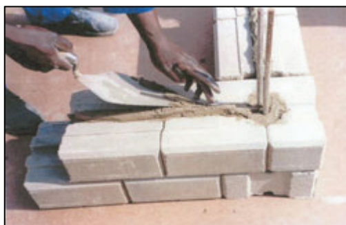
Figure 12: Hydraform interlocking blocks made from compressed stabilized earth ( http://www.hydraform.com )
