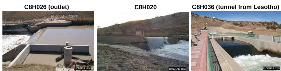
Figure 2.6 Photos of the flow stations in the Liebenbergsvlei catchments. These photos were obtained from the DWAF website ( http://www.dwaf.gov.za ).
