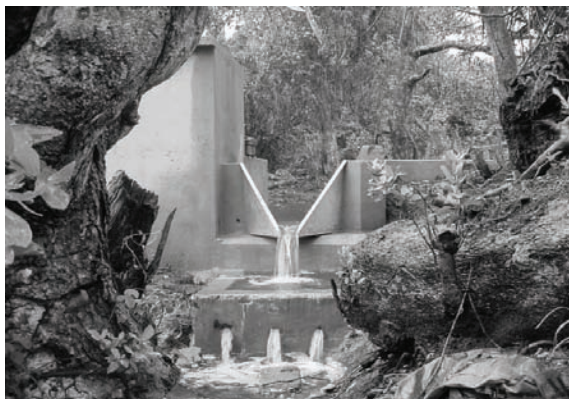
Photo 9. H-Flume of which the wing walls, foundation and ISCO housing were built.
