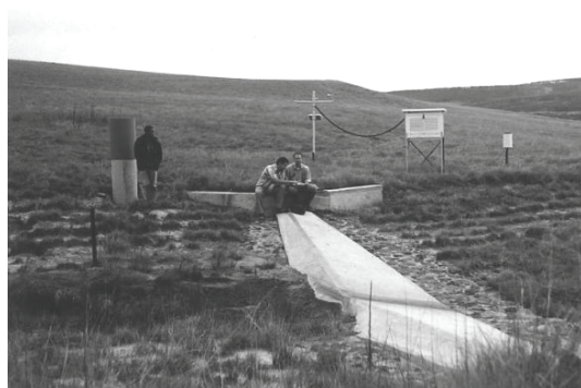
Photo 1. Mr Lentsoane at the upper weir at the Weatherley research catchment.
