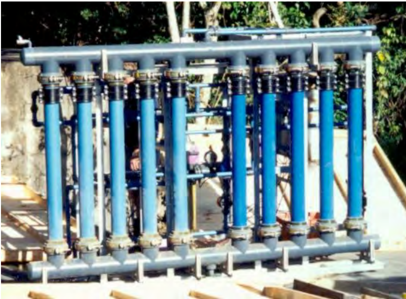
Figure 43: Connecting of 110 mm modules onto the 110mm top and bottom T-piece manifolds.
