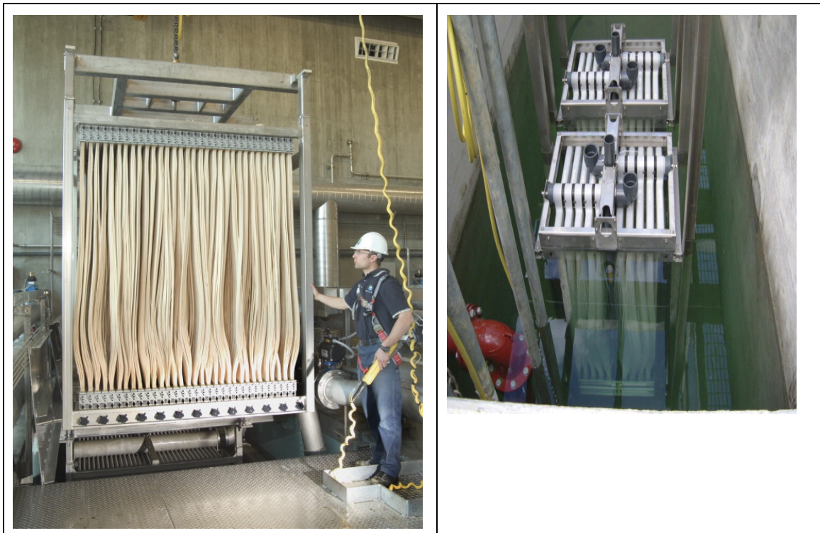
Figure 4:- Zeeweed® hollow-fibre module
