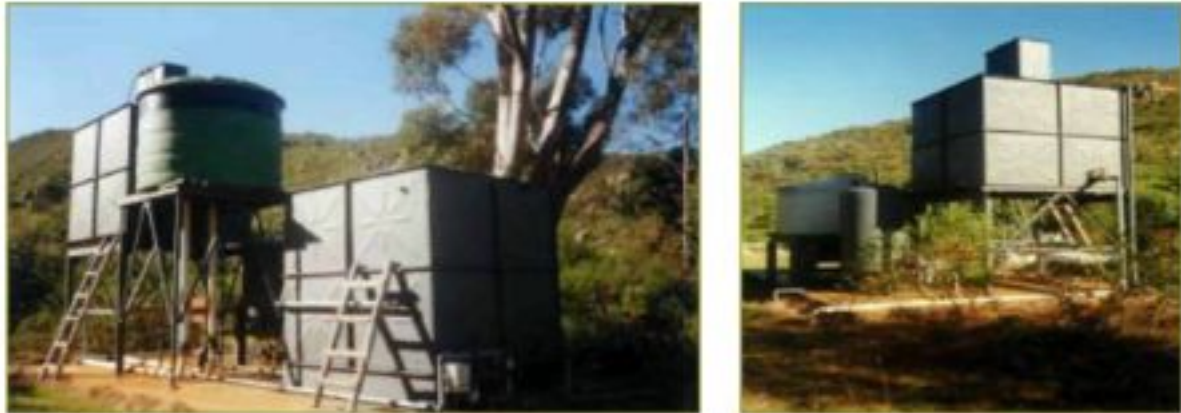
Figure 7.4: Plant "A" stabilisation/iron removal system
