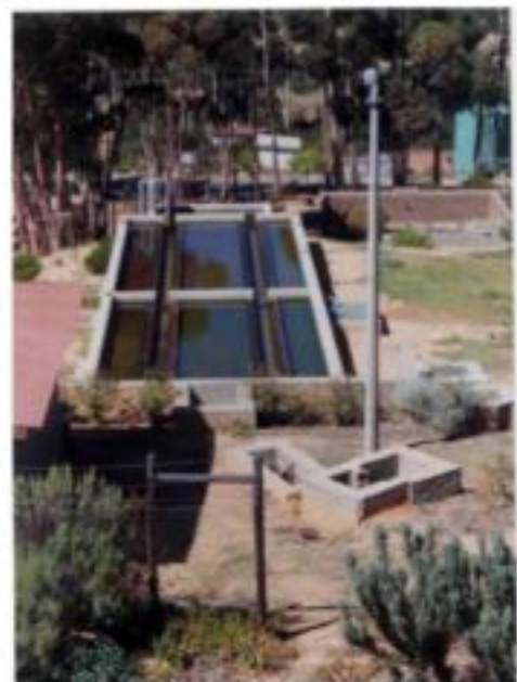
Figure 3.2: CSIR-type cylindrical design and alternative rectangular design limestone contact units
