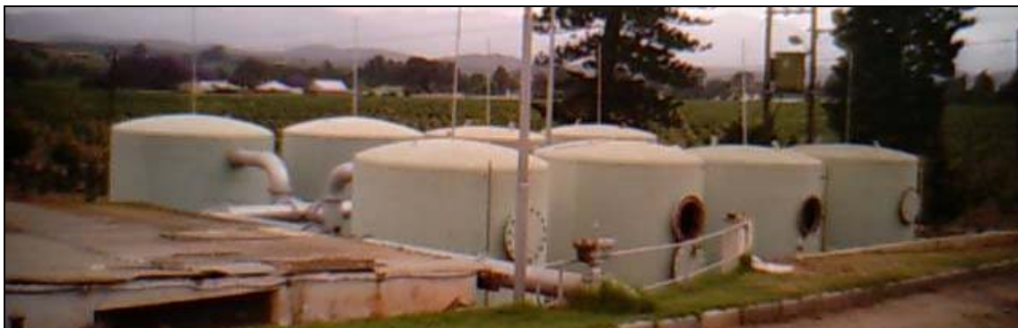
Figure 2-8: Pressure filtration units in Bonnievale – Western Cape
