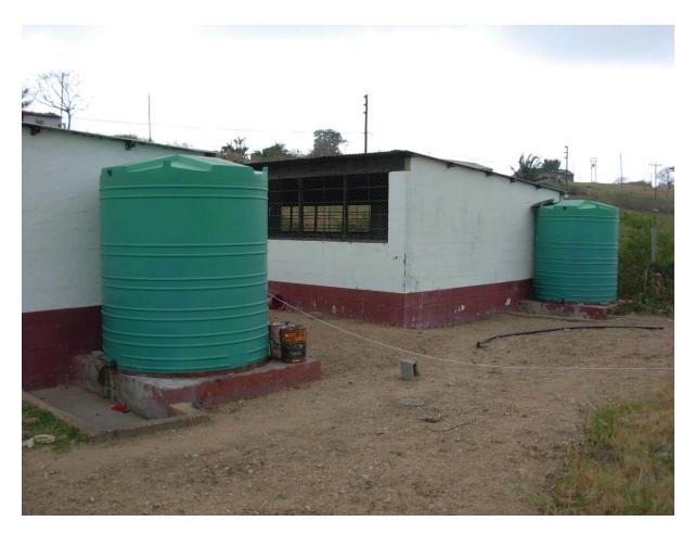
Figure 2.1: Micro-catchment rainwater harvesting and storage from rooftop rainwater
