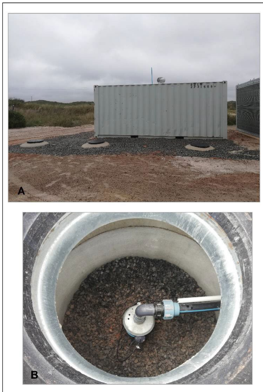
Figure 21. Positions of monitoring and injection boreholes fitted with manholes (A) and a look inside one of the injection boreholes (B).
