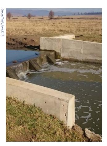
Concrete butress weir built during phase 1 of Working for Wetlands construction cycle.
