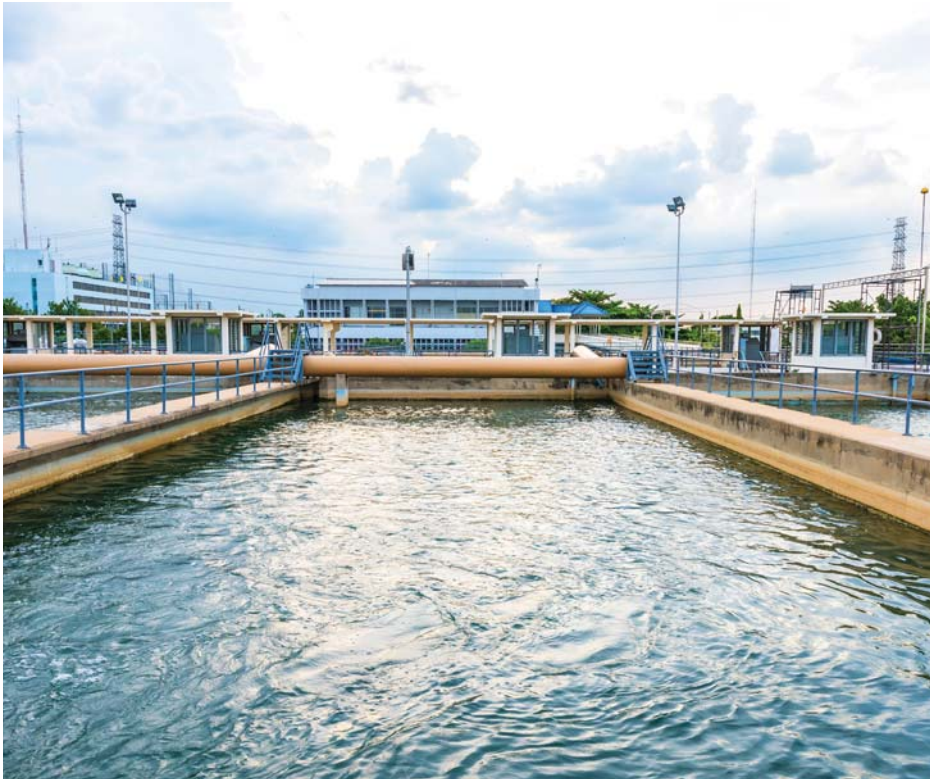
A typical rapid gravity sand filtration tank.
