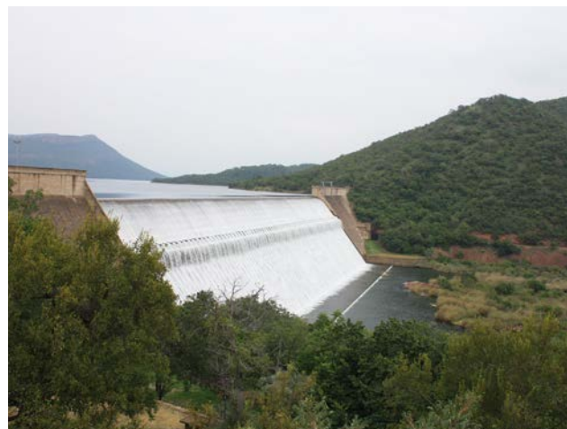
Loskop Dam in Mpumalanga irrigates an area of nearly 19 000 hectares via a 495-km long network of concrete-lined canals.
