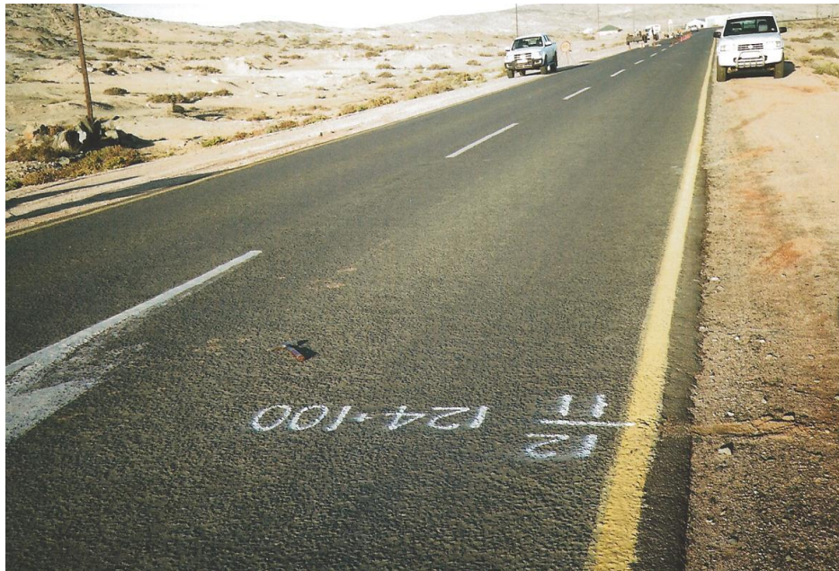
Figure A.6.5 29 March 2012 : Section 11 (Seawater in all layers), Left lane, view towards Aus. No current salt blisters, but scattered (Extent 3) small holes 50 mm diam. possibly representing broken blisters along centreline. Degree 1/Extent 5 map to star surface cracking over whole section. Similar cracking occurred over all the Lüderitz sections to a greater or lesser degree and extent including the control sections. West Control Section 14 (reseal at C priority) only marginally better than Section 11 (reseal at B priority).
