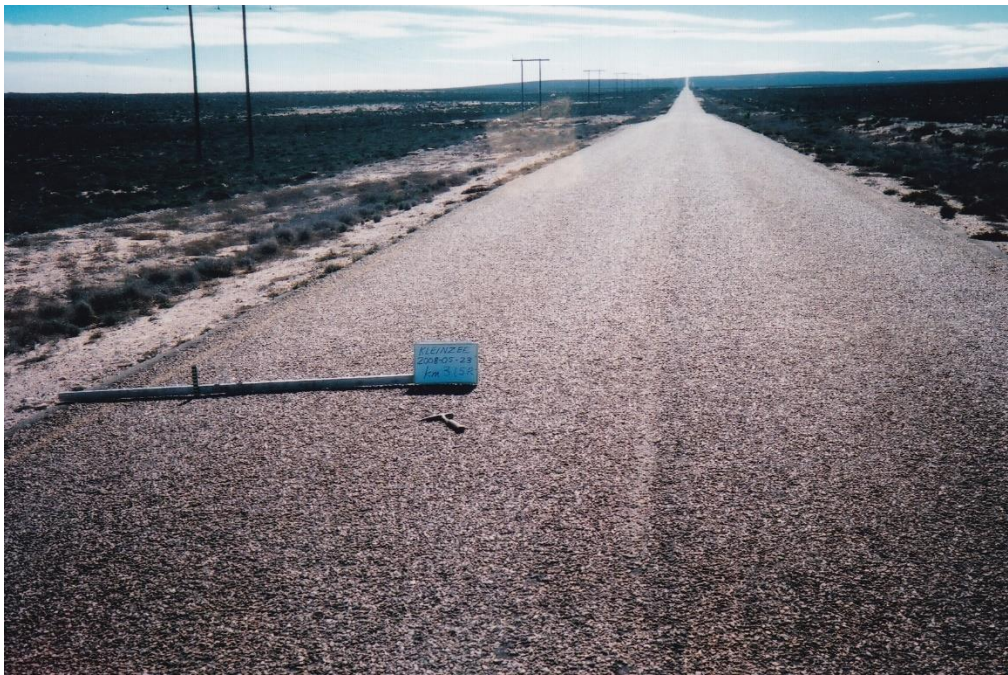
Figure A.8.7. Typical view of road towards Kleinzee after 28 years in May 2008 from km 31,5 over km 30-35 segment with mean base EC of 1,35 S/m and subbase EC of 0,79 S/m after compaction. General pavement condition good (and in 1986 and 1993); no edge breaking (0/5) (1/5 in 1993; edge drops about 10 mm; surfacing holes and patches 0/5 (1/5 in 1993); rutting about 10 mm (1/5); surfacing width 6,8 m.
