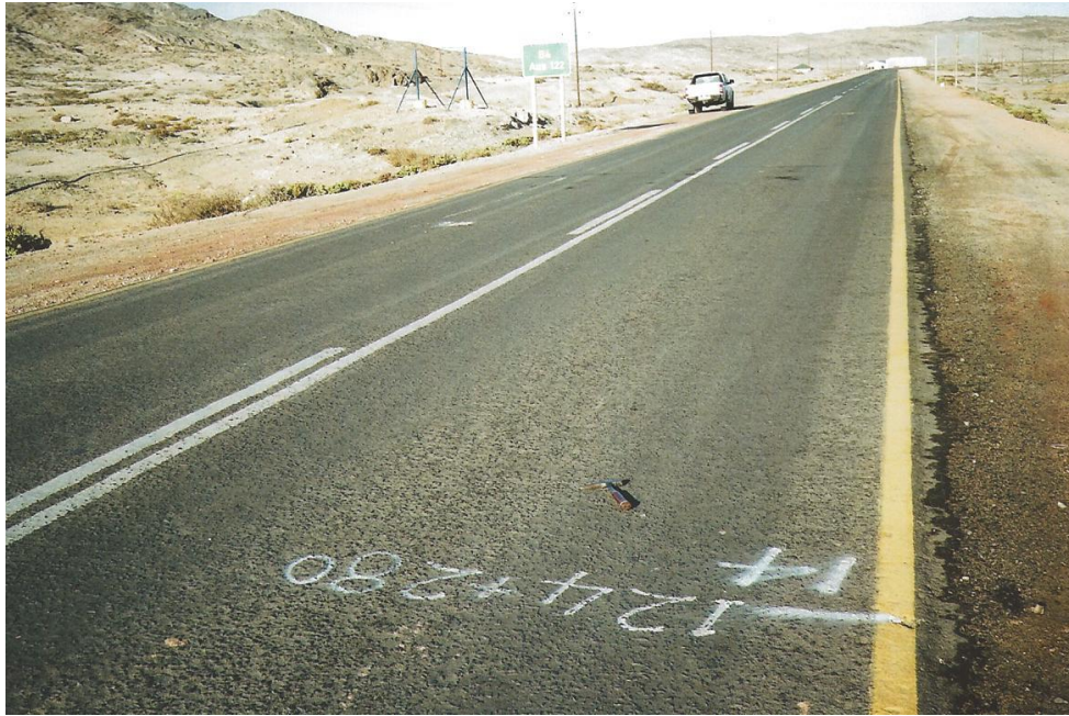
Figure A.6.4. (02 April 2012 after 36 years) : Section 14 (West control) at SV 124+280, left lane, view towards Aus. Best section on experiment. Degree 1/Extent 5 map to star surface cracking all over section. Full width slurry from approx. SV 124 + 261 to + 264. Rejuvenation or reseal at C priority recommended. Distinct wetness between wheelpaths on this and other sections after rain indicating permeable seal.
