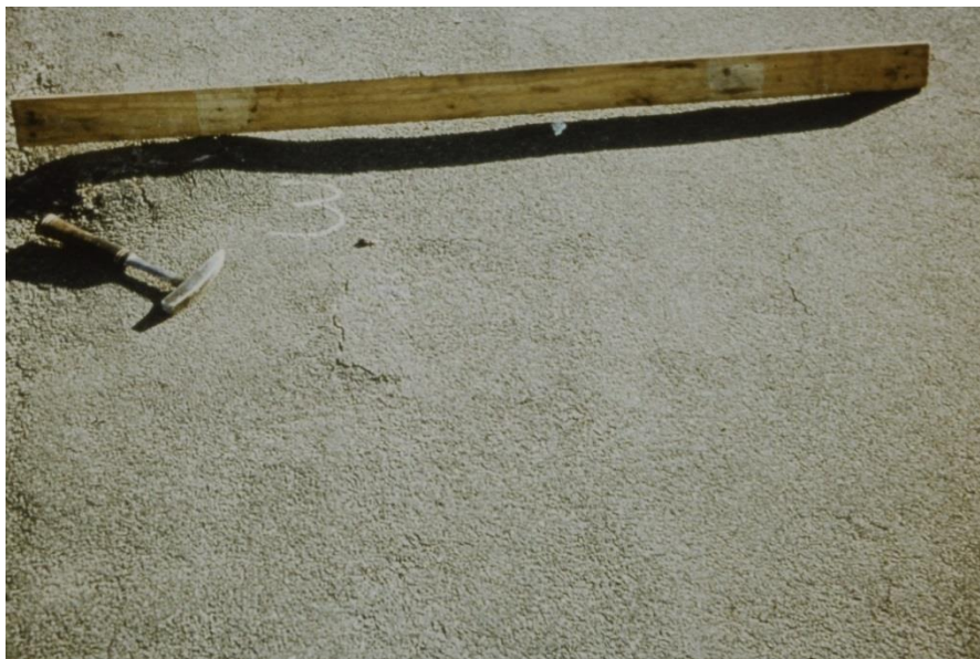
Figure 1.3: Closer view of very severe blister 30 mm high and 400 mm wide on old Walvis Bay airport.
