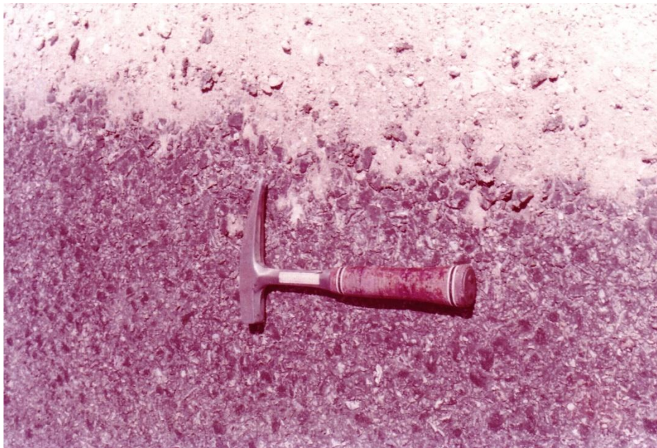
Figure A.8.5. Degree 1-3 edge fretting and surface shoulder looseness soon after construction.
