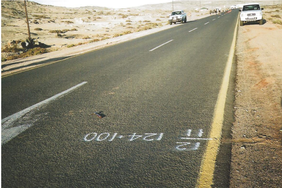
Figure 4.4: After 36 years without a reseal : Section 11 (seawater in all layers), view towards Aus.
