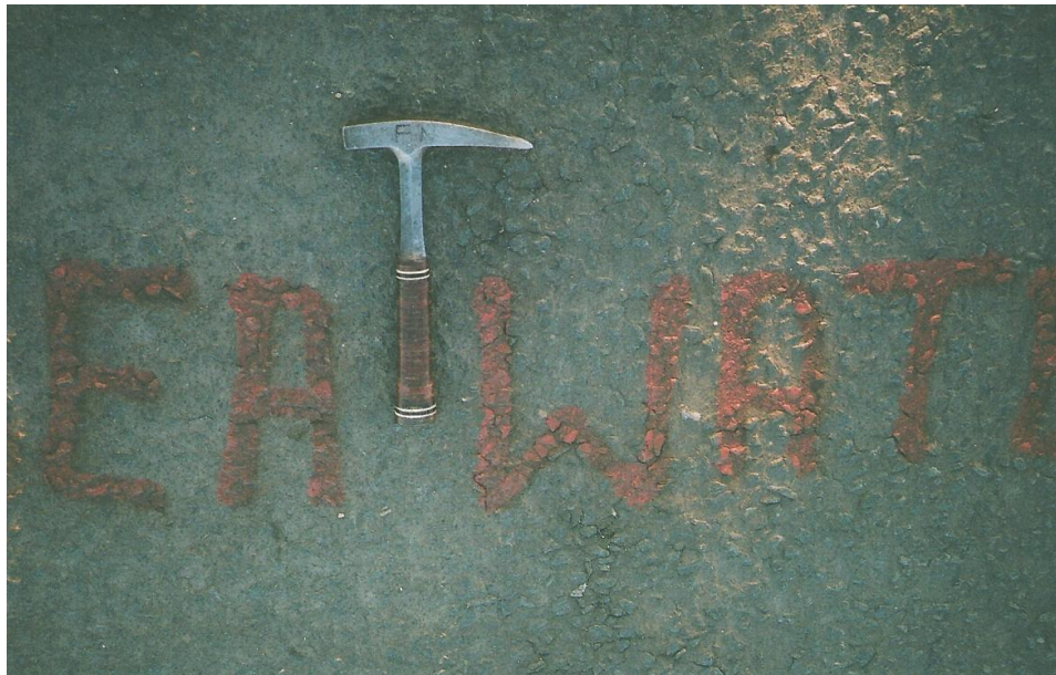
Figure A.6.3 (29 March 2012: Section 11 (Seawater G3 at SV 124 + 070, Right midlane). Close-up view of worst cracking on section (Degree 1/Extent 5 random to star surface, averaging 50 mm length at 100 mm spacing).
