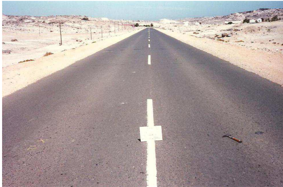
Figure A.6.1: (03 Feb. 1991): Section 10 (5% gypsum + seawater), view towards Lüderitz. No salt blisters, but Degree 1/Extent 5 map to star surface cracking, especially in right lane.
