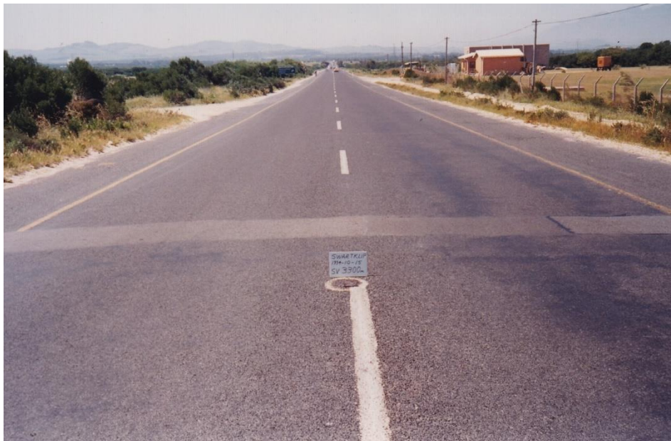
Figure 4.3: View towards Faure interchange of seawater crushed stone base section after 19 years in 1994.
