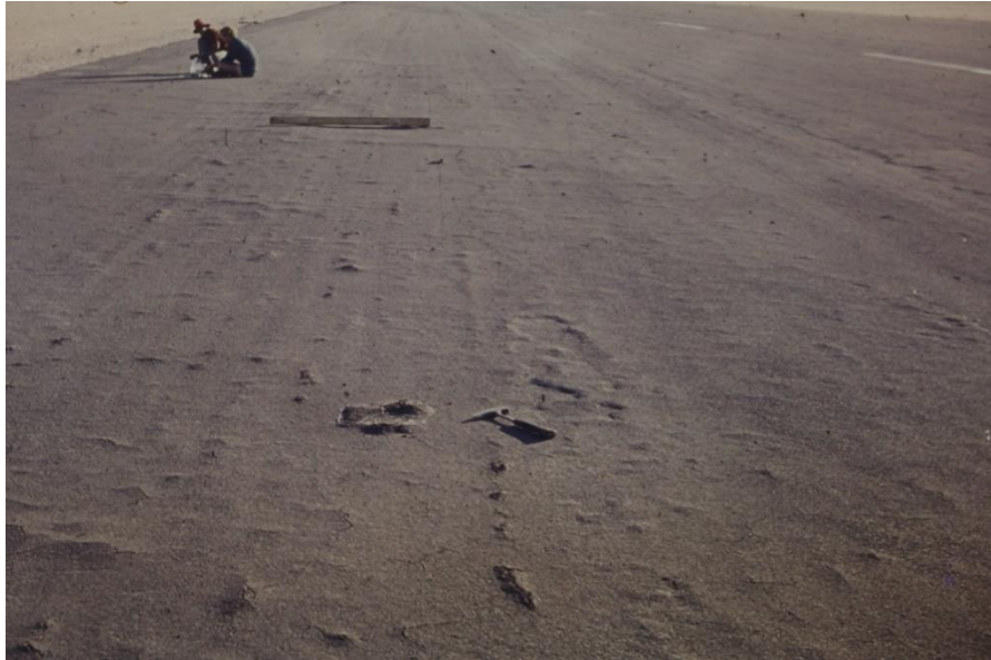
Figure 1.2: Very severe blistering and cracking of triple seal on old Walvis Bay airport due to crystallisation of halite (NaCl) in the upper base due to use of salt water in subbase (Netterberg, 2015)
