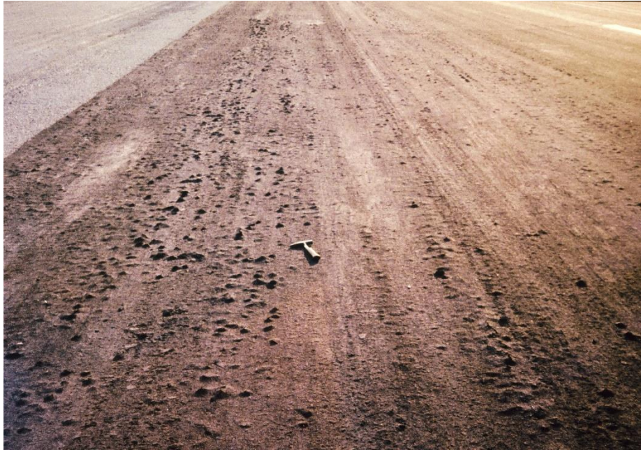
Figure 2.2: Severe blistering of 13 mm Cape seal on Sua Pan airport due to crystallisation of halite in upper base from salt compaction water used in subbase and lower layers (Netterberg and Bennet, 2004).
