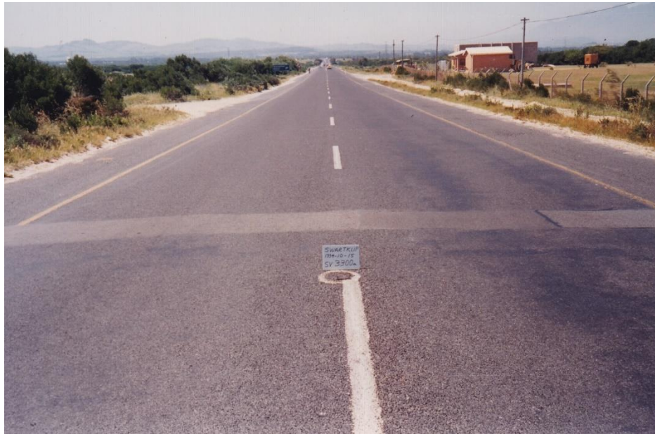
Figure A.4.4. View towards Faure interchange of seawater crushed stone base section after 19 years in 1994. Section SV 3 300 marker plate on centreline placed in 1975 shown ringed
