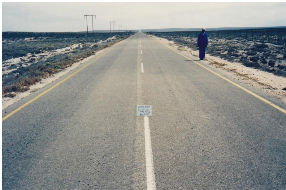
Figure A.8.6. Typical view of road towards Kleinzee in good condition after 28 years in February 1992 from km 31,0 over km 30-35 segment with mean calcrete base EC of 1,35 S/m and subbase EC of 0,79 S/m after compaction. Small (20 mm) Degree 4 / Extent 5 black bleeding spots. Overall pavement condition good in 1992/3, 1986 and 2008; edge breaking Degree/Extent 1/5 (4/5 in 1986); number of surfacing holes/patches 1 204 (i.e. 241/km) as at April 1985 (1/5 in 1993, none (0/5) in 2008).
