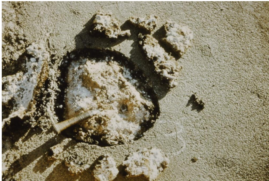
Figure 1.4: On opening the blister much white halite (NaCl) was evident and the full depth of the G3 crushed stone base course could be excavated by hand.
