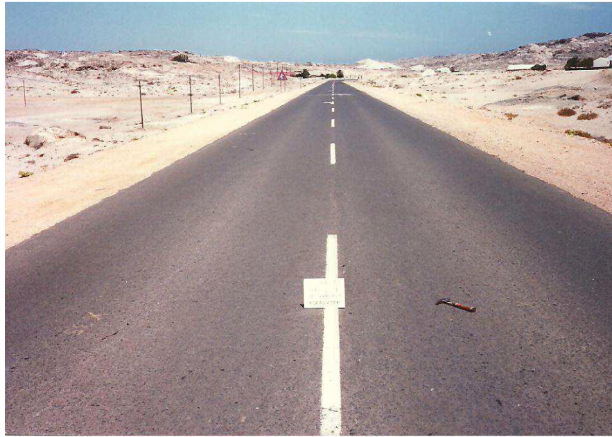
Figure A.6.2 (03 Feb. 1991). Section 11 (Seawater in all layers), view towards Lüderitz. No salt blisters, but Degree 1/Extent 5 map to star surface cracking. Similar cracking occurred on all Lüderitz sections including the controls.
