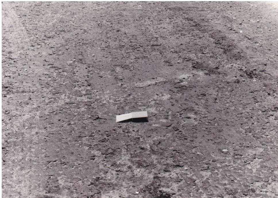
Figure A.4.1. Prime damage on seawater calcrete base
