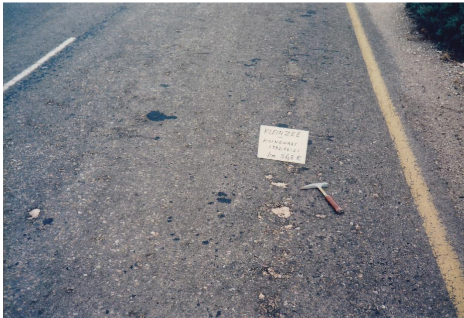
Figure A.8.2. Showing small white surfacing holes (“potholes”) and black bleeding spots, white calcrete chips, and a few black patched holes in seal at km 56,8R after 12 years in February 1992 (cumulative total of 342/km holes and patches around this point up to April 1985). Mean EC of km 55-60 segment of calcrete base 0,74 S/m and subbase 1,26 S/m after compaction; Degree/Extent of holes and patches in 1993 3/2; overall pavement condition in 1992/3 fair, (good in 1986 and 2008).
