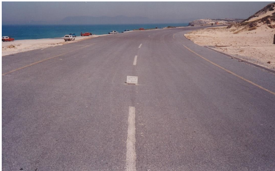
Figure A.4.3. View towards Muizenberg of SV 200-300 seawater calcrete base section after 19 years in 1994
