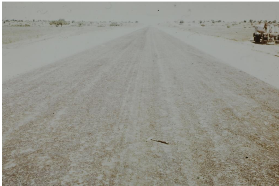
Figure 1.1: Typical mild surface disintegration of primed base course due to crystallisation of salt from brackish compaction water in the base course.
