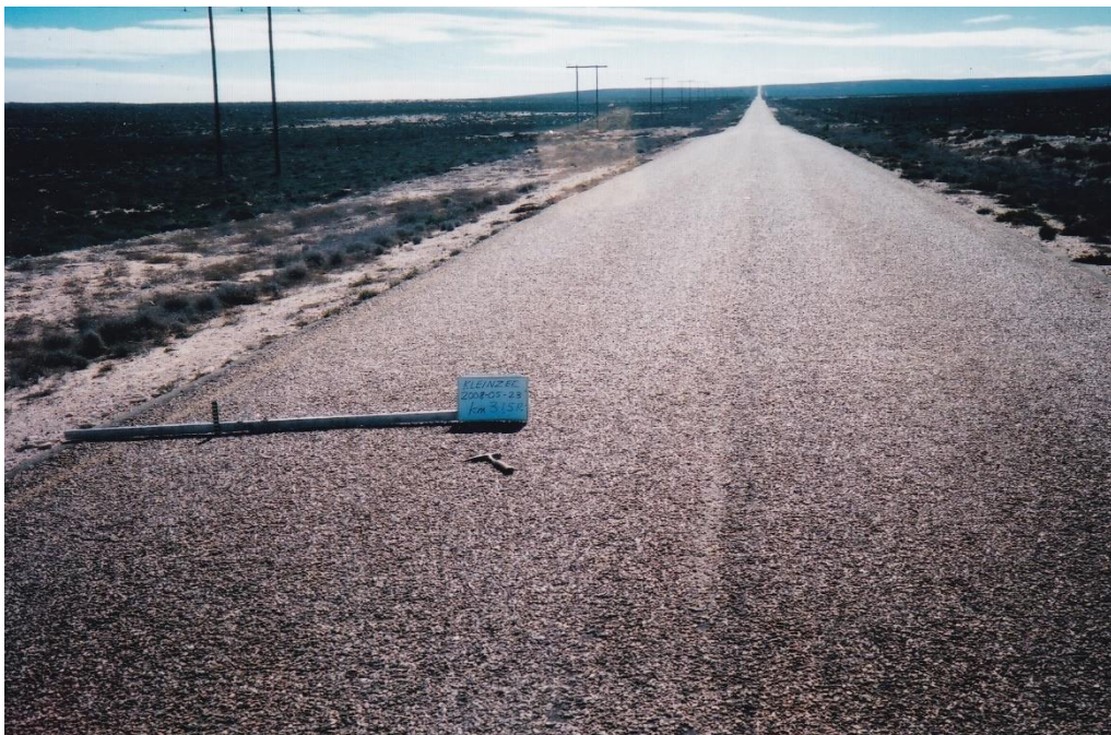
Figure 4.5: Typical view towards Kleinzee after 28 years in May 2008 from km 31,5 over km 30-35 segment with mean base EC of 1,35 S/m and subbase EC of 0,79 S/m after compaction with seawater.
