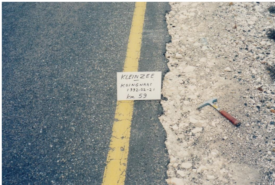
Figure A.8.4. Showing Degree 2-3 edge breaking at km 59 after 12 years in February 1992 and coarseness and tightness of calcrete gravel base and localised strip of partly disintegrated white calcrete chips (cumulative total of 273 holes and patches/km around this point up to April 1985). Mean EC of km 55-60 segment of base 0,74 S/m and subbase 1,26 S/m after compaction; Degree/Extent of edge breaking 3/3 (3/5 in 1986); overall pavement condition in 1992/3 fair (good in 1986 and 2008).
