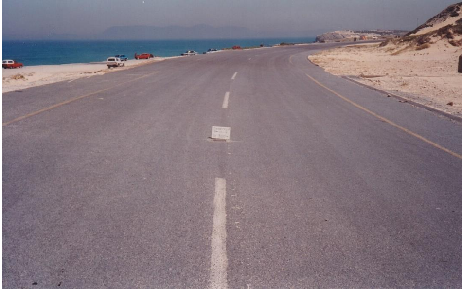
Figure 4.2: View towards Muizenberg of SV 200-300 seawater calcrete base section after 19 years in 1994.
