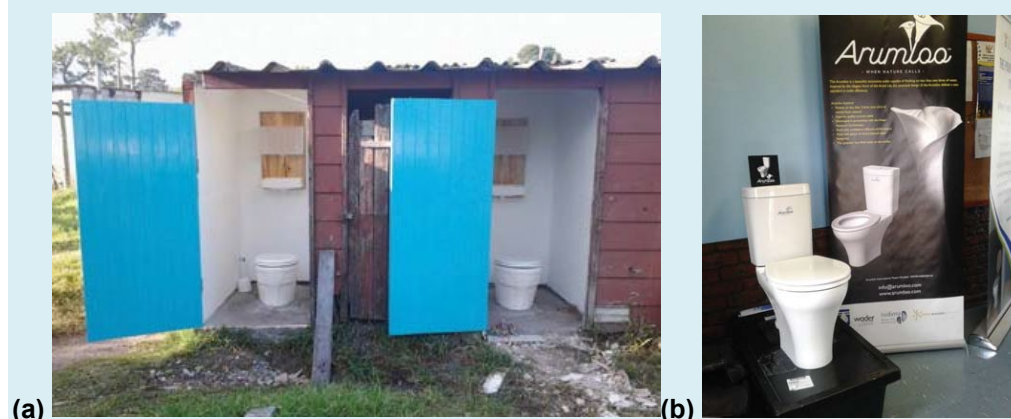
Figure 10: Example of innovations in end-user installation materials in the Wet WASH value chain showing (a) a Pour Flush Toilet and (b) the Arum Micro-flush toilet (taken from Amis and Lugogo (2018))
