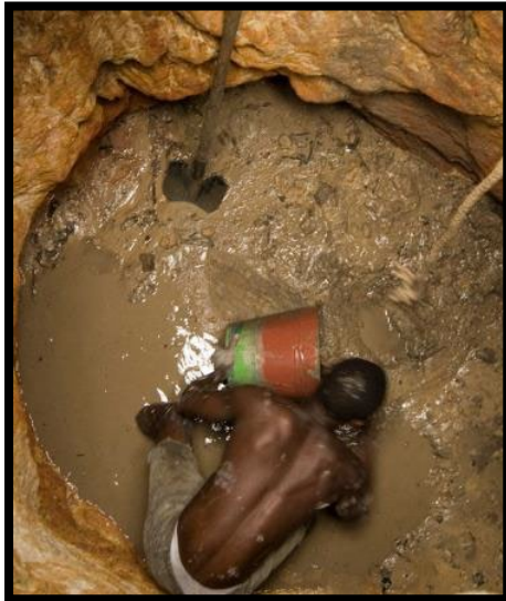
Figure 13. Digging of a water well by hand
