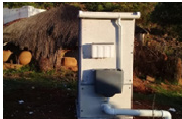
Figure 5. Installation of low flush units. Community members were trained in sanitation planning and hygiene education, and local community members were employed through a process facilitated by Tsogang Water and Sanitation.
