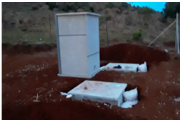
Figure 5. Installation of low flush units. Community members were trained in sanitation planning and hygiene education, and local community members were employed through a process facilitated by Tsogang Water and Sanitation.
