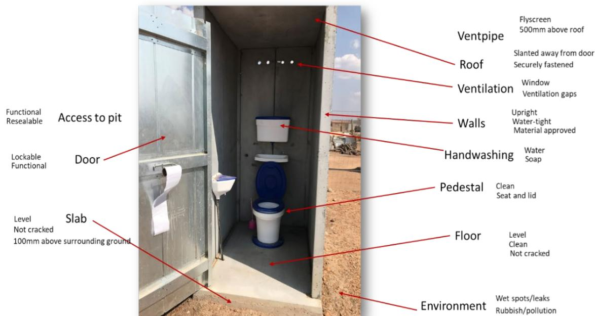
**Figure 28: Some elements of sanitation to be recognised by computer vision**
