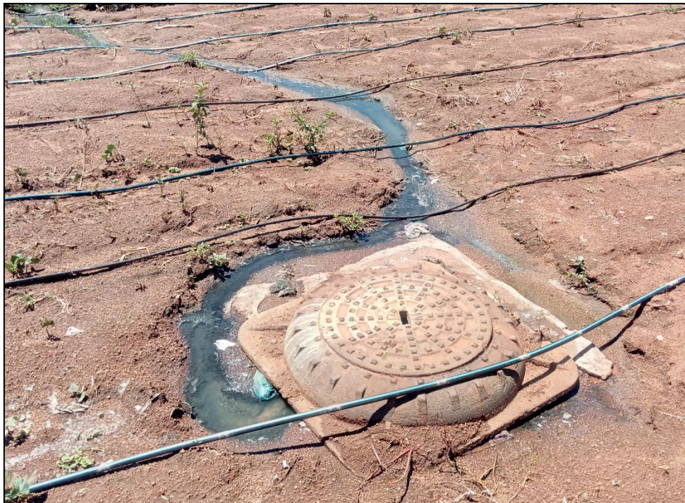
Figure 3-5: Raw sewage leaking into the Rooiwal Agri-park fields in January 2019
