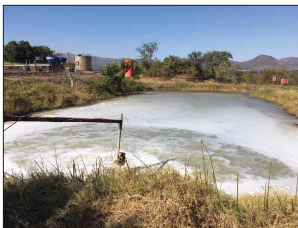
Figure 6.2: Anaerobic lagoons used at industrial unit 3103.2
