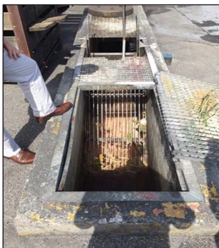
Figure 6.8: Screen filter used in industrial unit 3013.12 (prior to neutralisation treatment)
