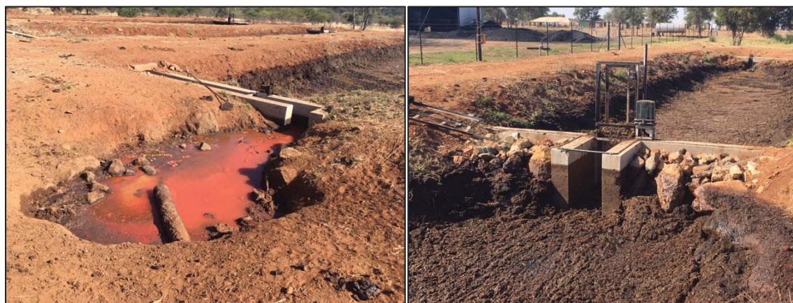
Figure 6.4: Settling dams with moving screen filter at industrial unit 3103.5 (angle 2)
