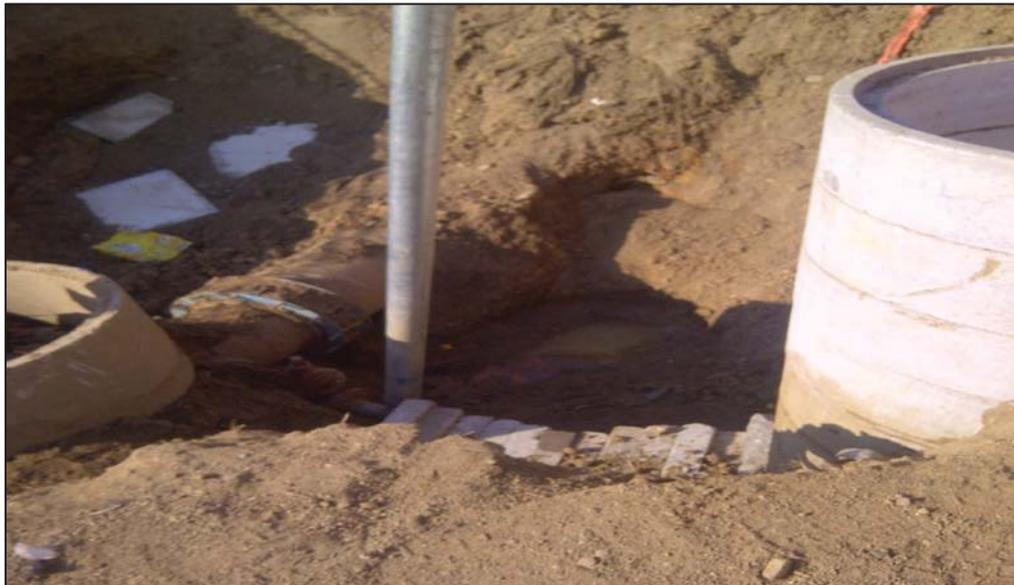
**Figure 3-4: Water pipeline thrust block supported by a sewer manhole**
