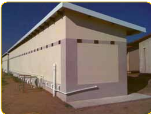
New Toilet blocks at Thandaza High School
