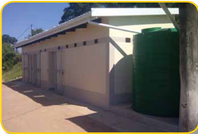
Newly built toilet blocks at Sizimesele Primary School
