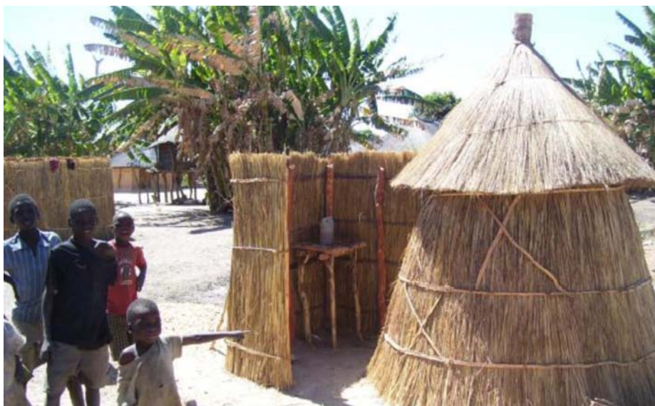
Standard latrine constructed in rural areas using local resources
