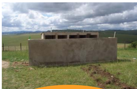
Building being re-plastered
