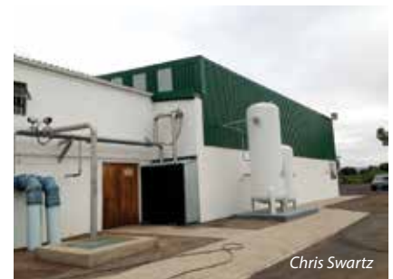
The Beaufort West reclamation plant.
