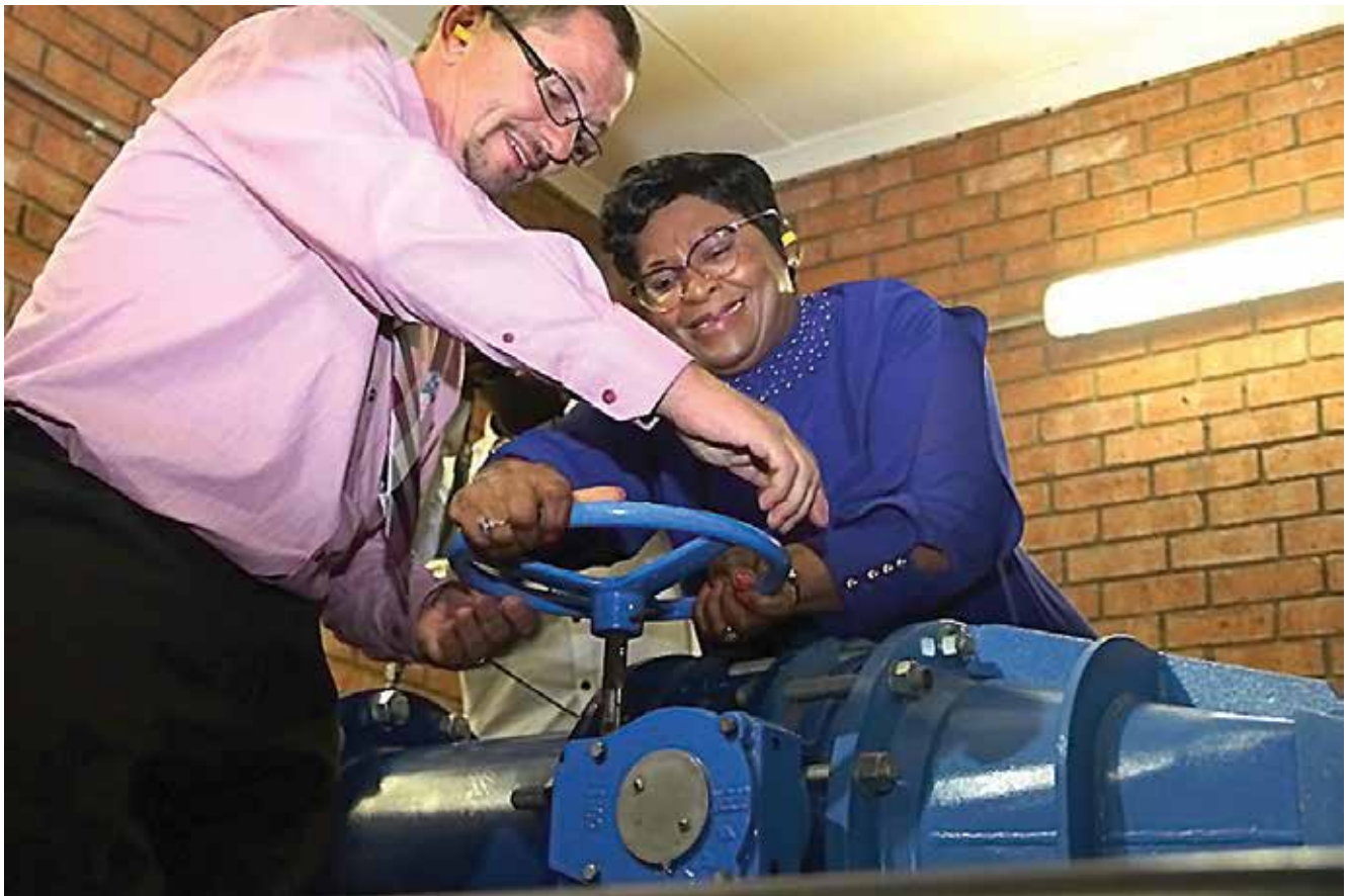
Bloemwater electrical technician, Jacques van Delft, assists Minister of Water and Sanitation, Nomvula Mokonyane, to open the valve at the conduit hydropower facility at Brandkop reservoir.
