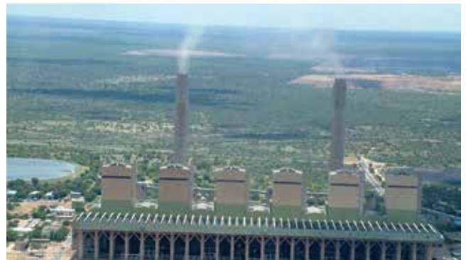
Matimba power station is one of many power stations in South Africa located in a water scarce area.
