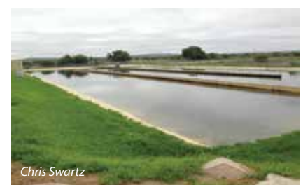
Treated effluent from Beaufort West's wastewater treatment works passes through maturation ponds before entering the reclamation plant.
