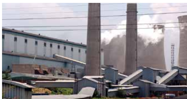
Grootvlei is one of the previously mothballed power stations that have been returned to service.
