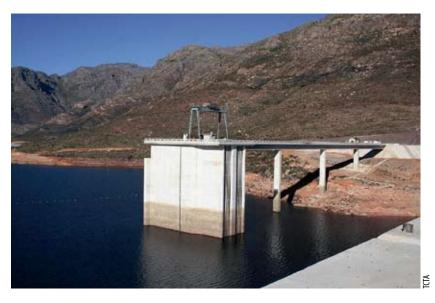
The Berg River Dam intake tower is divided into two sections. The north section is a dry shaft (well) equipped with multi-level inlets, pipes and valves, which provides the facility for drawing water into the Cape Town supply system and provides for low flow environmental releases.
