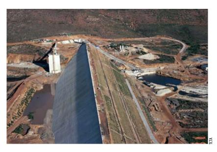
The Berg River Dam is a concrete-face-rockfill dam type. The dam is 65 m high, 990 m wide and 220 m in width. The gross storage capacity of the dam is 130 million m<sup>3</sup>. The outlet works have been designed to release both low flows and high flows with provision for a peak release of up to 200 m<sup>3</sup>/s. This makes it the first dam in South Africa in which provision is made for flood releases for environmental purposes.
