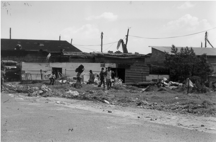
Figure 4 Damage in Intabazwe (Goliger and Van Wyk, 1999)
