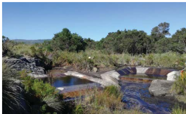
Completion of work to address two headcuts just upstream of the main site – SUCCESS!
