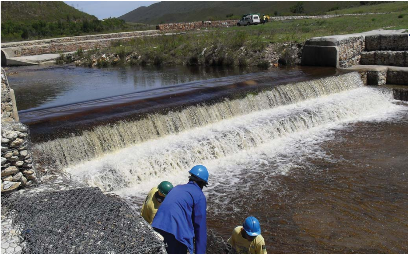
In an effort to protect the last remaining peatlands and palmiet wetlands of the Kromme River in the Eastern Cape's Langkloof, Working for Wetlands has funded a number of costly erosion-control weirs.
