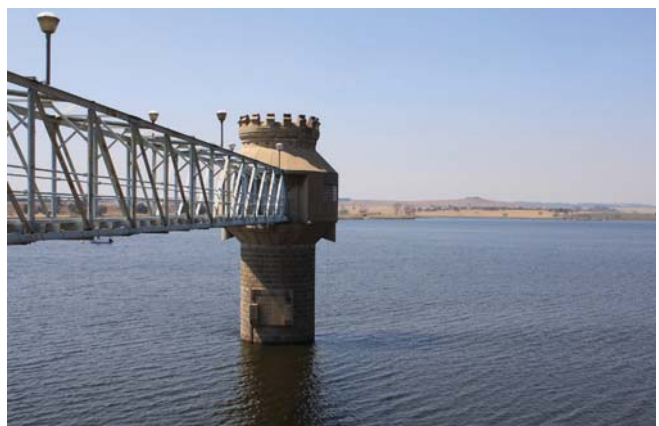
The concrete outlet tower feeds water to the adjacent purification plant.
