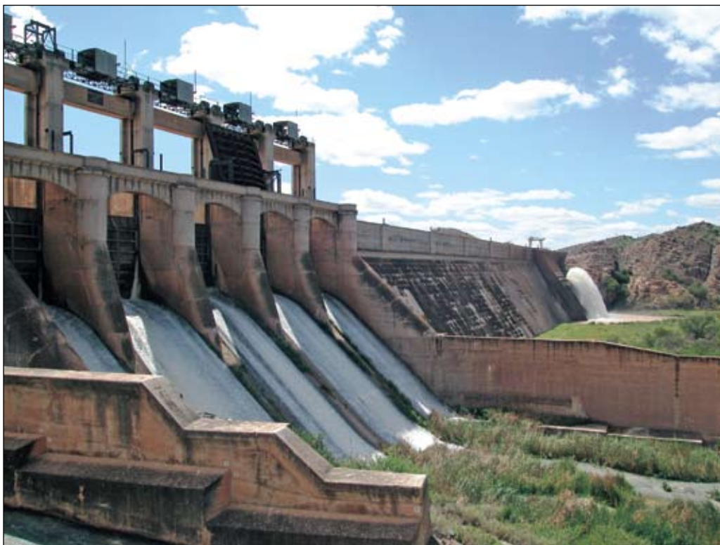
The dam wall has two spillways with control gates – the main spillway and an auxiliary spillway. Near the left abutment is the river outlet system with a number of release valves.
