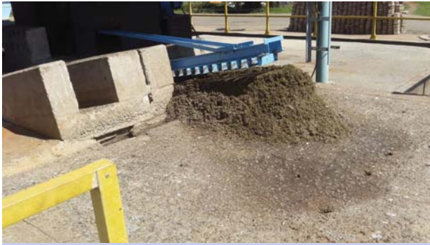
When blocked sewers were cleared with storm water the plants received a large amount of grit.
