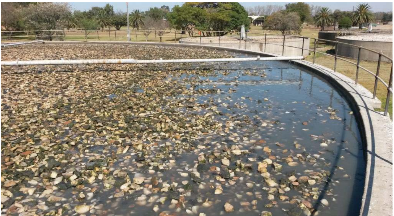
Ponding on biofilter due to blockages.
