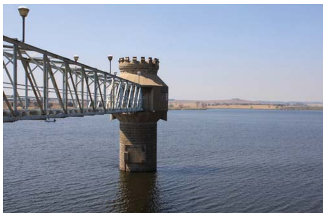
The concrete outlet tower feeds water to the adjacent purification plant.
