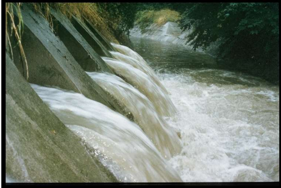
Combined sewer overflow (CSO)
