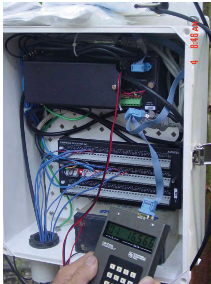
Figure 5.11 A view of a datalogger and multiplexer wired to only four of the potential 12 probe sets per multiplexer and 24 probe sets per datalogger.
