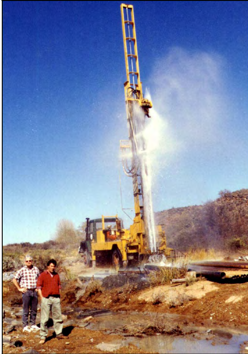
The editors at an exploration site on a dolerite sill in the Victoria West District, during the drilling of an artesian borehole with a drillstem yield of 80 \ell/s
