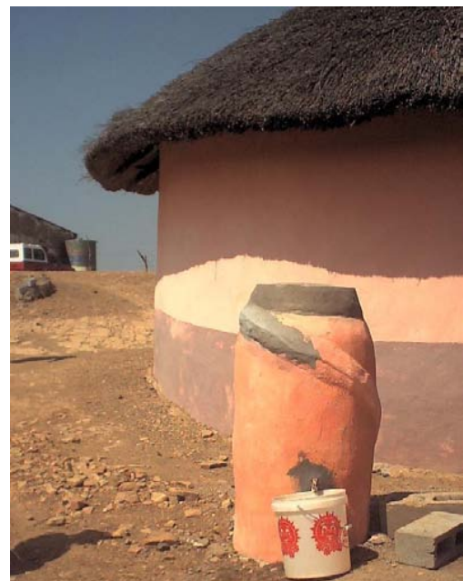
A tank at Nondayana. (Note plaster seal on lid and encased inlet pipe)
