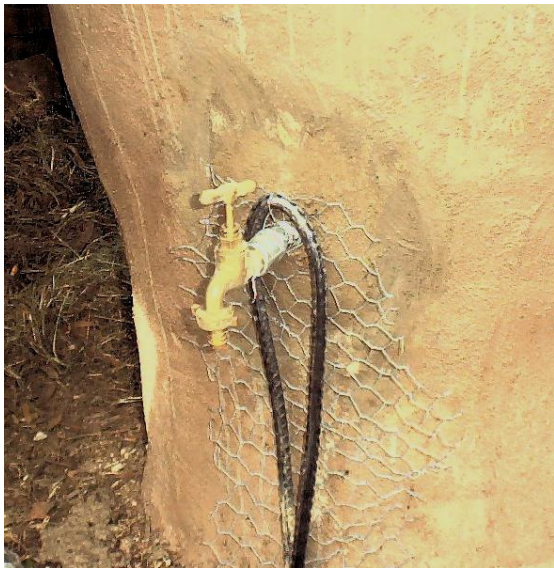
Reinforcement of the tank outlet tap.
