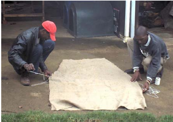
The hessian is first sewn into bags for the stand and tank.
