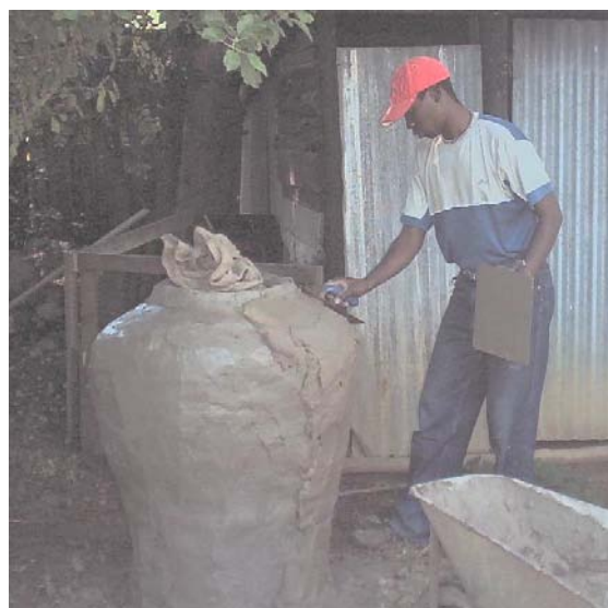
A second layer of plaster is applied.
