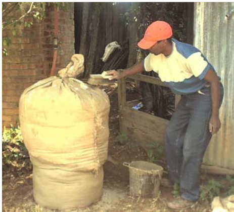
A cement slurry is applied to ensure binding of the plaster.
