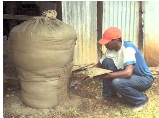
Plaster is applied to the outside.
