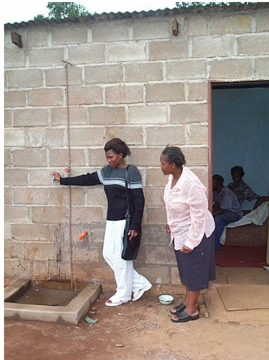
Figure 4 – Typical Bypass of Household Tank
