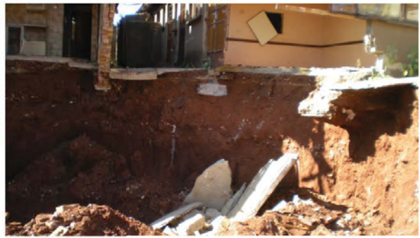
(b) Khutsong, 10 m increased to 30 m diameter sinkhole, affected two other houses (30 May 2017).
