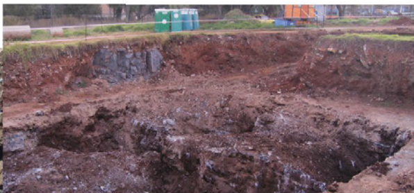
(f) Pier foundation of rail system (City of Tshwane, © MA Dippenaar 2010).
