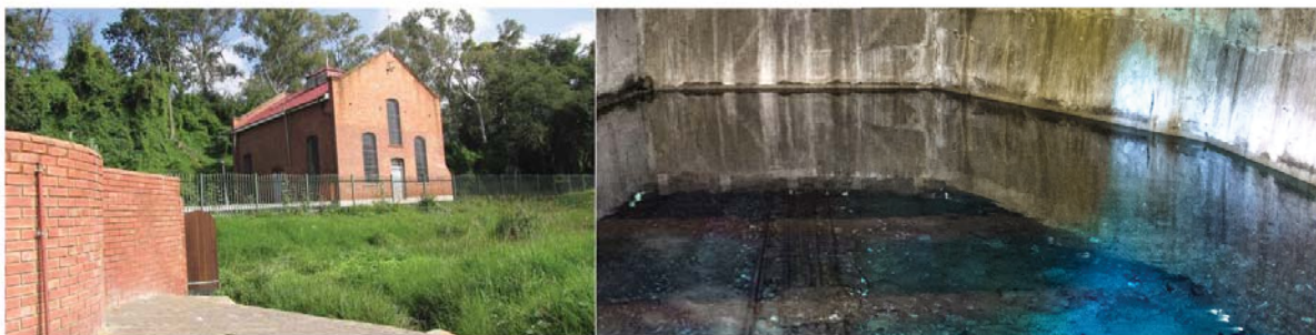
(b) View of the collection chamber and pumphouse, as well as view inside the collection chamber of Lower Fountain spring partially supplying Pretoria (2017).
