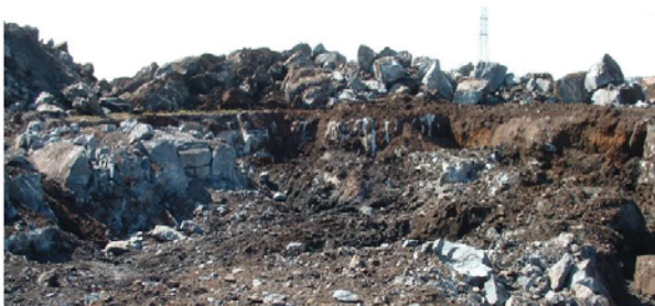
(e) Removal of pinnacles for foundations (City of Tshwane, © JL van Rooy 2004).
