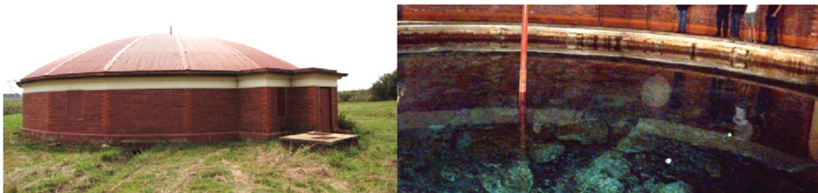
(c) View of the collection chamber, as well as view inside the collection chamber of Grootfontein spring partially supplying Pretoria (2017).
