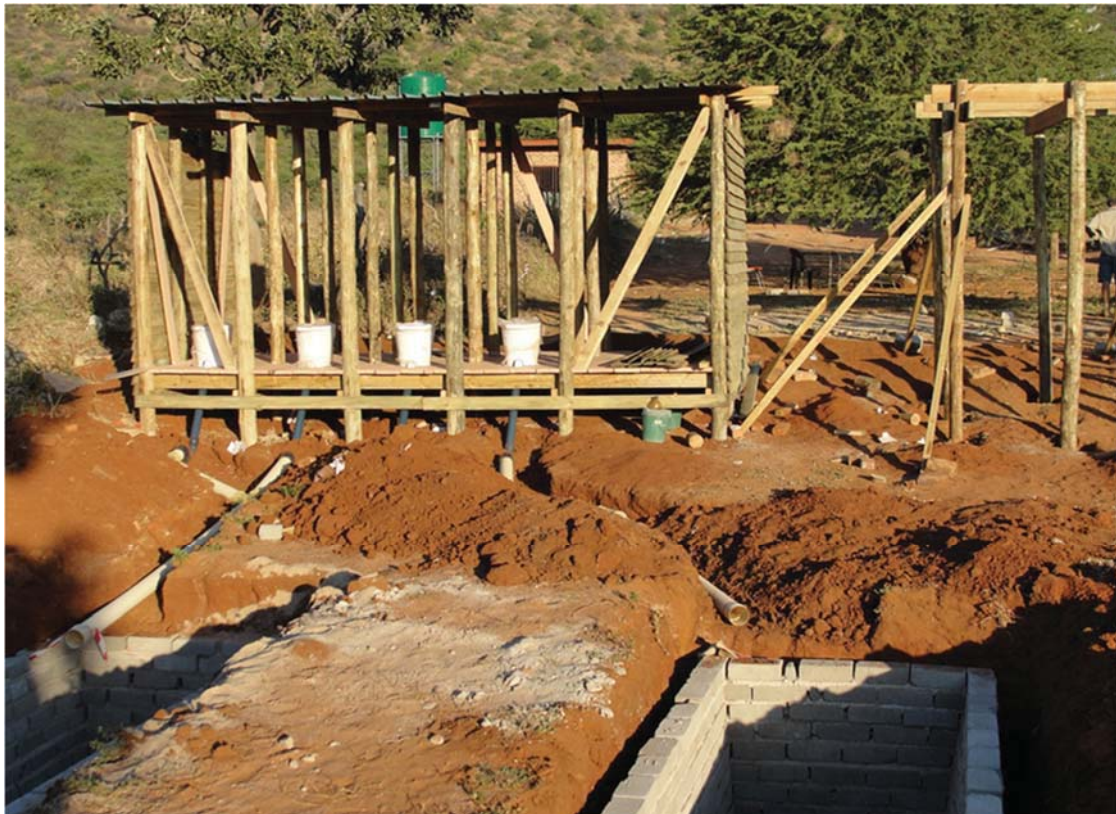
Figure 8: Construction of the pour-flush toilets in a school in Limpopo (Still, 2015)
