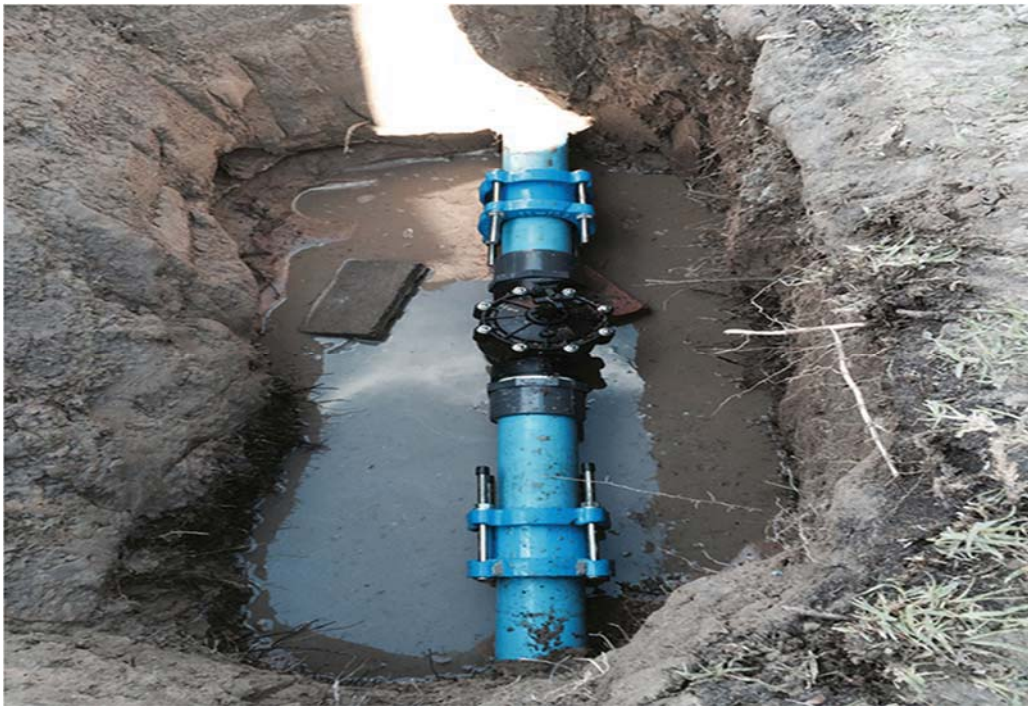
Figure 26 : Image of an installed Aquatrip (source: Splash Plumbing, n.d.)
