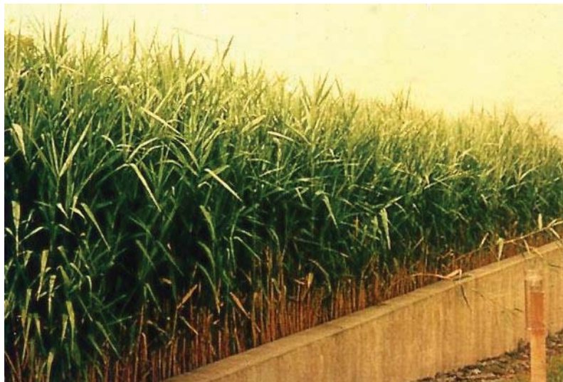
Figure 11: Sludge drying bed with emergent plants.
