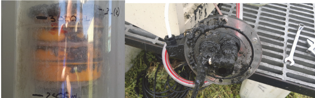
Figure 70: Accumulation of sludge on top of the flow switch, and on the bottom of the reactor. Note the reduced, black, 'rotten' nature of the sludge.
