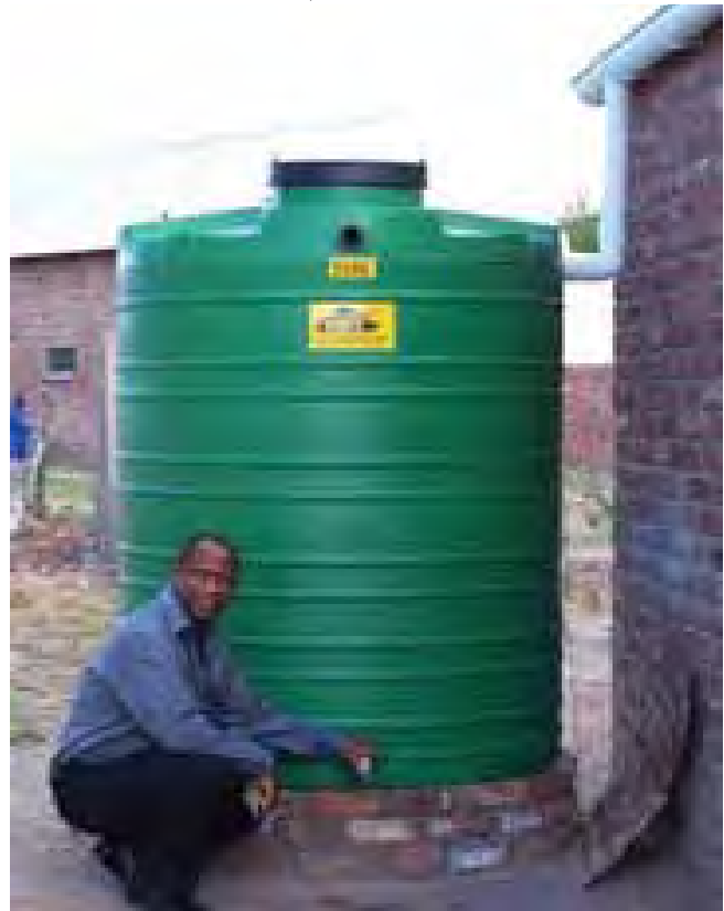
Figure 1: Water tank used in harvesting rainwater
