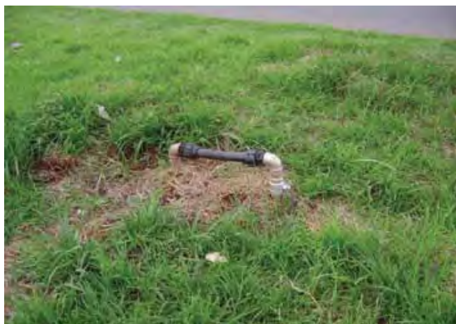
Figure 2: Unmetered connection
