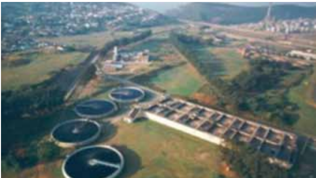
Figure 1: Durban Water Recycling Plant
