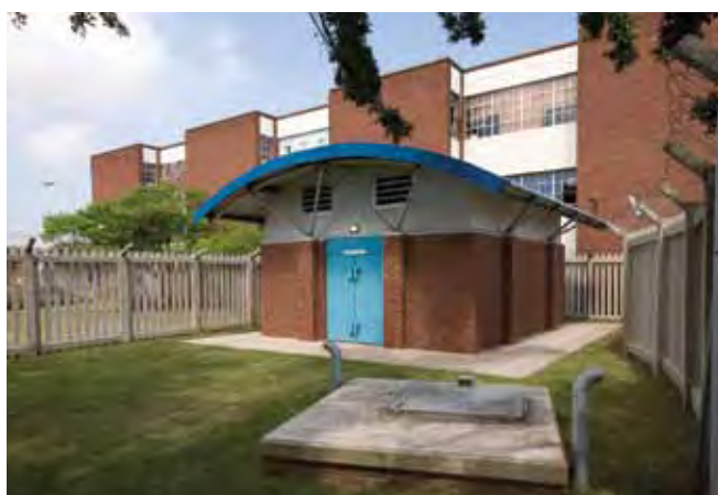
Figure 2: PRV and meter chamber
