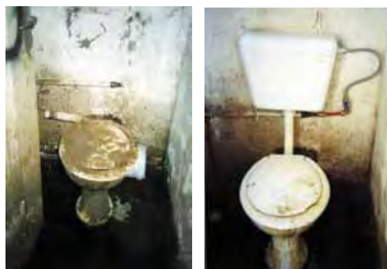
Figure 3: Toilet that was repaired as part of the project
