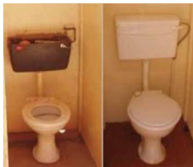
Figure 1: before and after repairs
