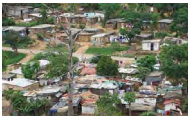
Figure 2: Informal Settlement without access to basic sanitation
