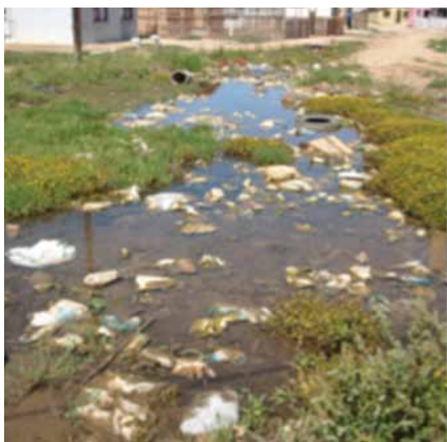
Figure 2: Burst Pipe located during investigation in residential area
