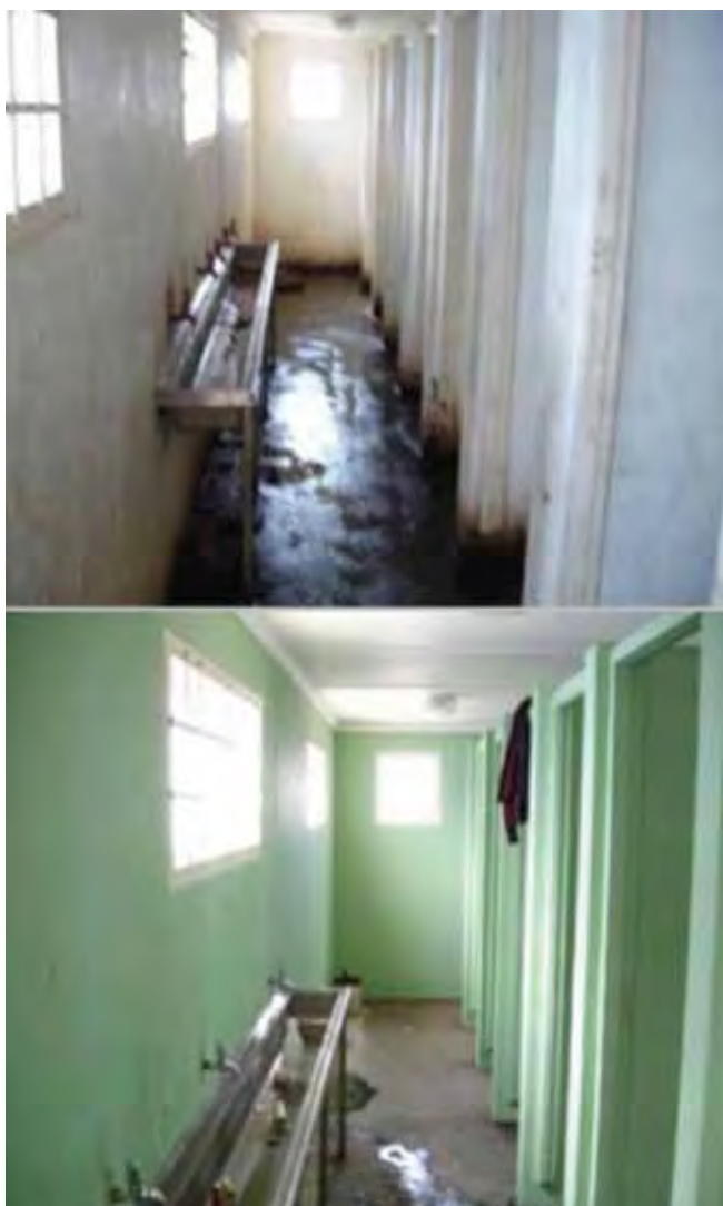
Figure 2: If the budget allowed, then ablution facilities were painted including structural repairs
