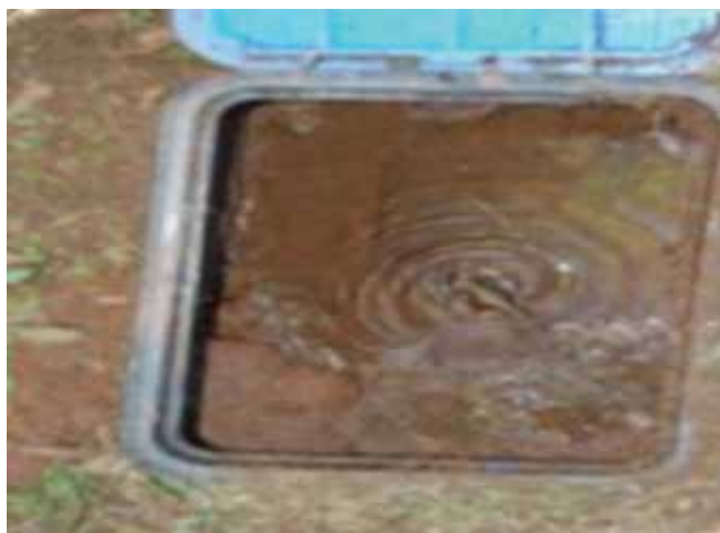
Figure 2: Leaking meter
