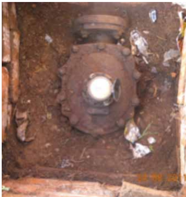
Figure 4: Example of old/non-functioning water meter identified for replacement
