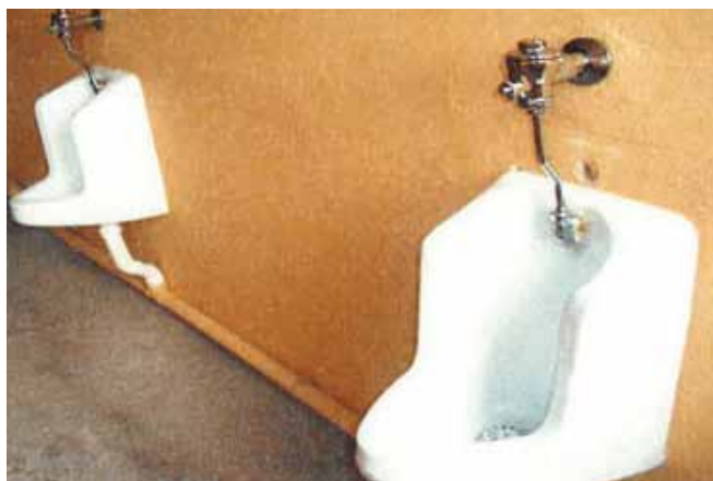
Figure 4: (After) Retrofitted manual flushing urinals
