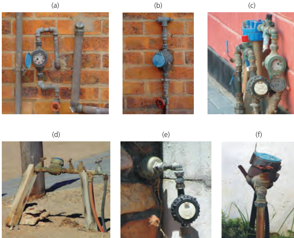
Figure 5-2 Examples of incorrect meter installations
