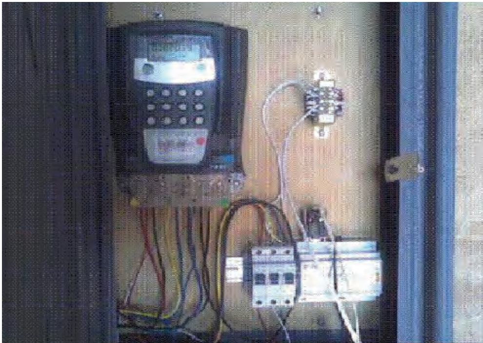
Plate 3.11: An installed ElectroFlo water and energy meter
