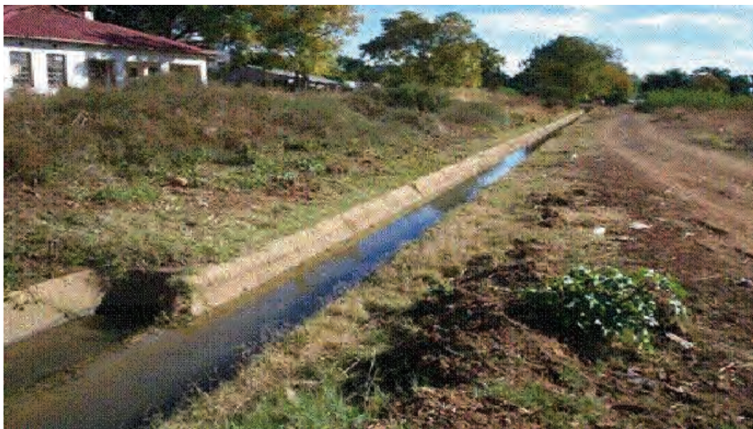
Plate 3.12: Grass cleared along the main canal in Block 4A
