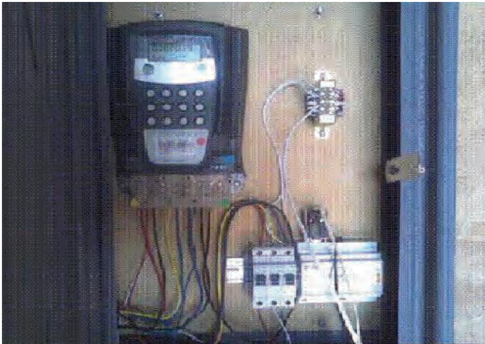
Plate 3.11: An installed ElectroFlo water and energy meter
