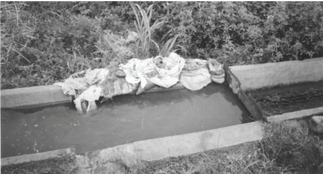
Plate 3.6: Lack of maintenance of canals threatens the sufficiency of one of the most critical natural resources at Tugela Ferry; water
