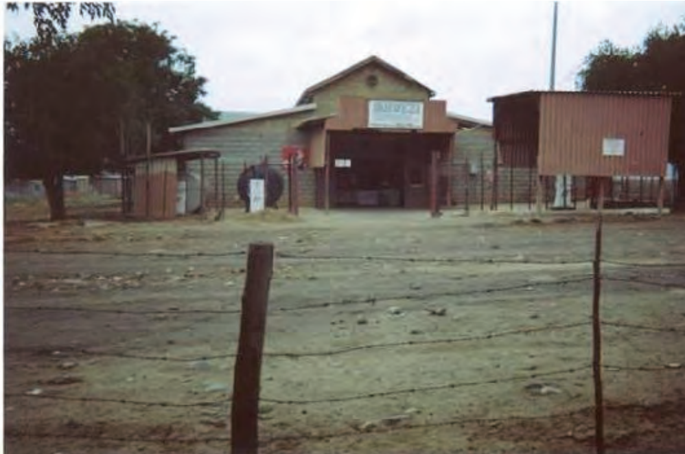
Plate 3.2: The defunct Ikhwezi Cooperative building which is currently used for general dealership (Photograph taken in 2005)
