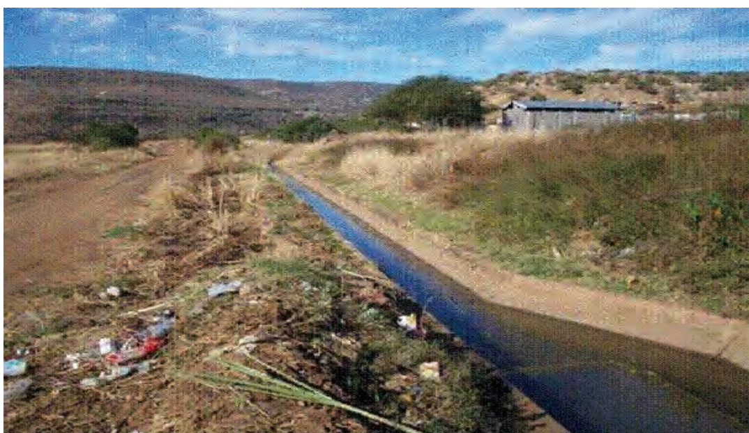
Plate 3.13: Debris removed from the canal
