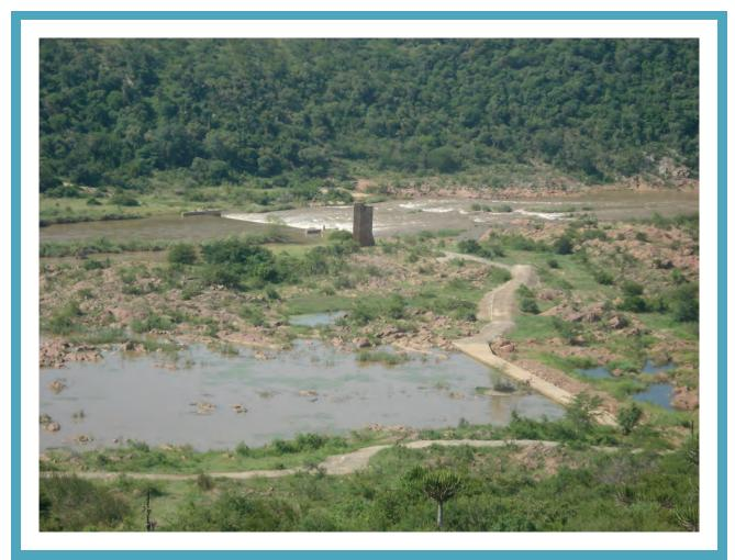
Photo 7: The gauging weir monitoring flows between South Africa and Mozambique at Ressano Garcia. The international agreement is that a minimum of 2.6 m <sup>3</sup>/s should flow over the weir
