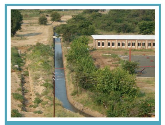
Photo 13: Middle Letaba Dam has an off-take canal feeding agriculture schemes but the use from this canal is to a large extent unregulated and a serious regulation problem
