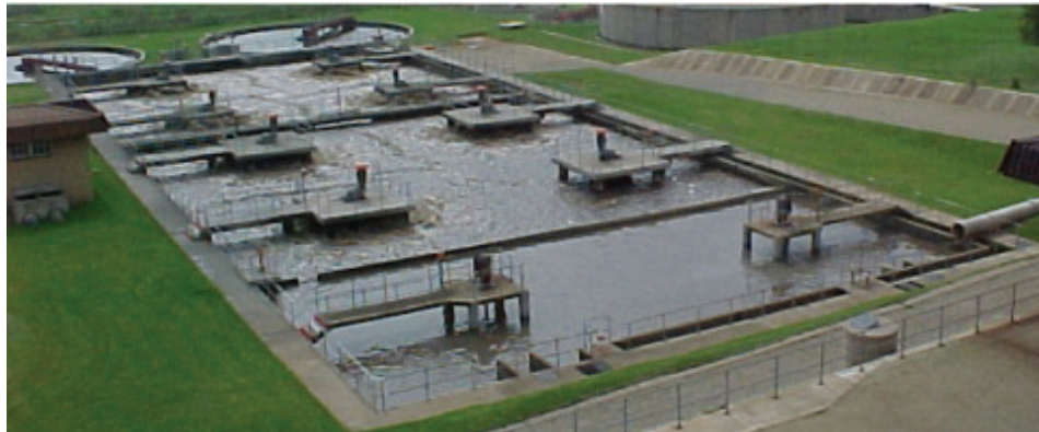
FIGURE 7.1.1: Typical activated sludge reactor basin (eWISA)
