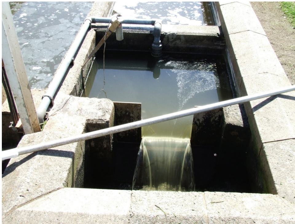
FIGURE 3.1.2: Example of a rectangular weir
