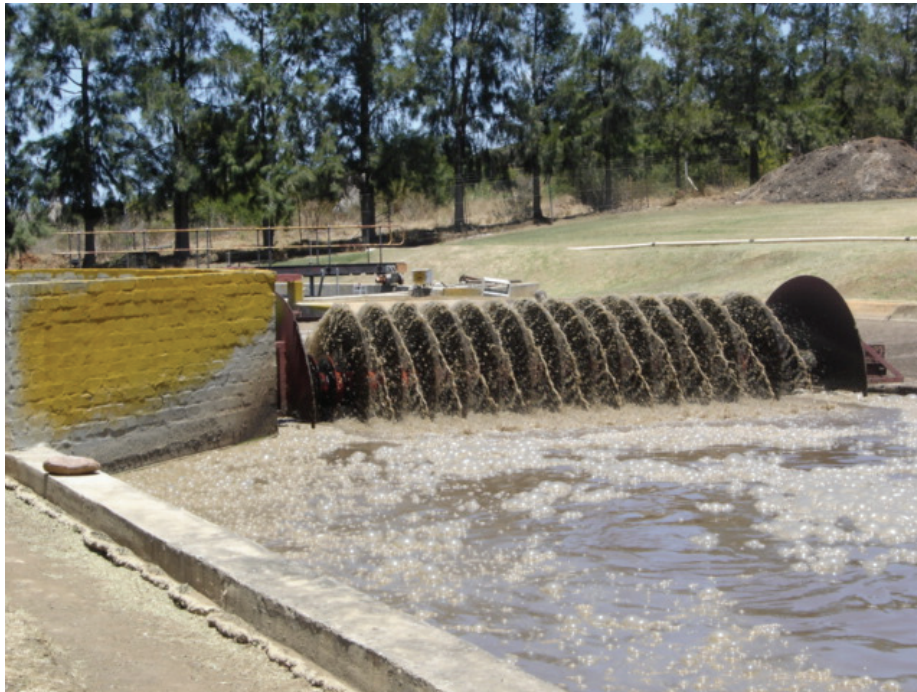
FIGURE 8.3.1: Rotating bio contactor
