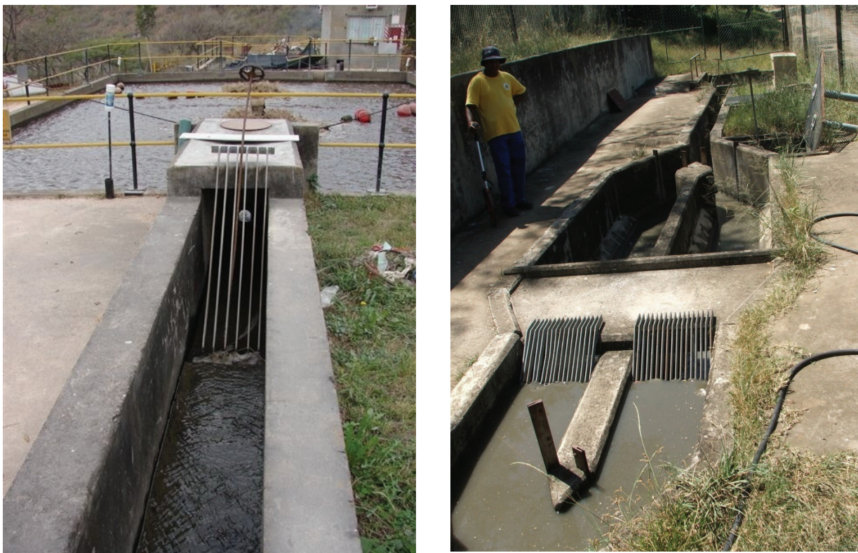
FIGURE 3.2.1: Typical coarse screens
