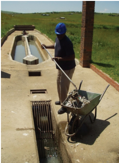
FIGURE 3.2.2: Manual cleaning of screens
