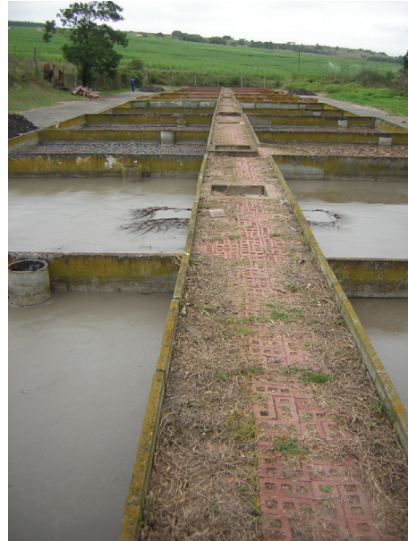
FIGURE 9.4.1: Typical sludge drying beds (eWISA)
