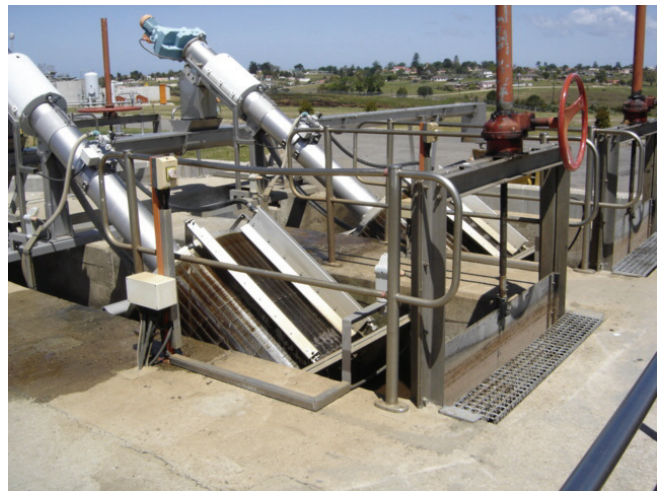
FIGURE 3.2.3: Mechanically raked screens (eWISA)
