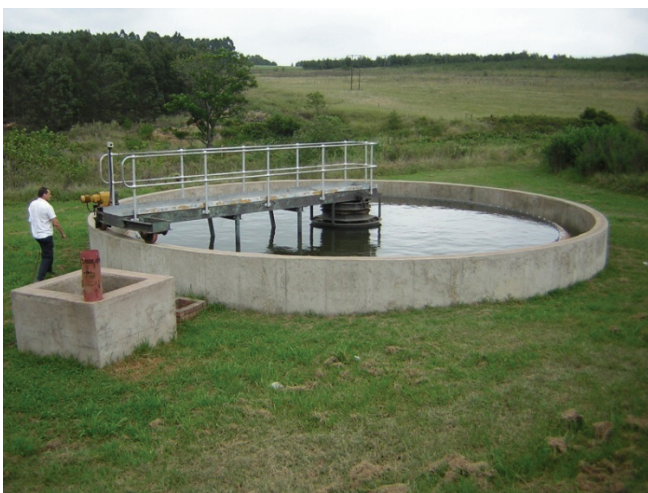
FIGURE 6.3.2: Typical secondary sedimentation tanks
