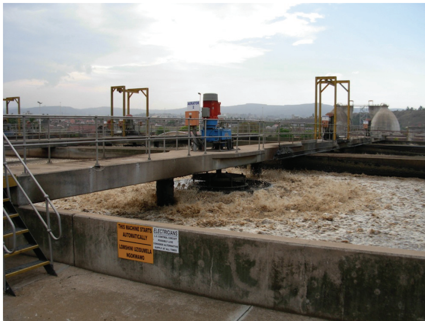
FIGURE 7.5.1: Typical bridge-mounted surface aerator
