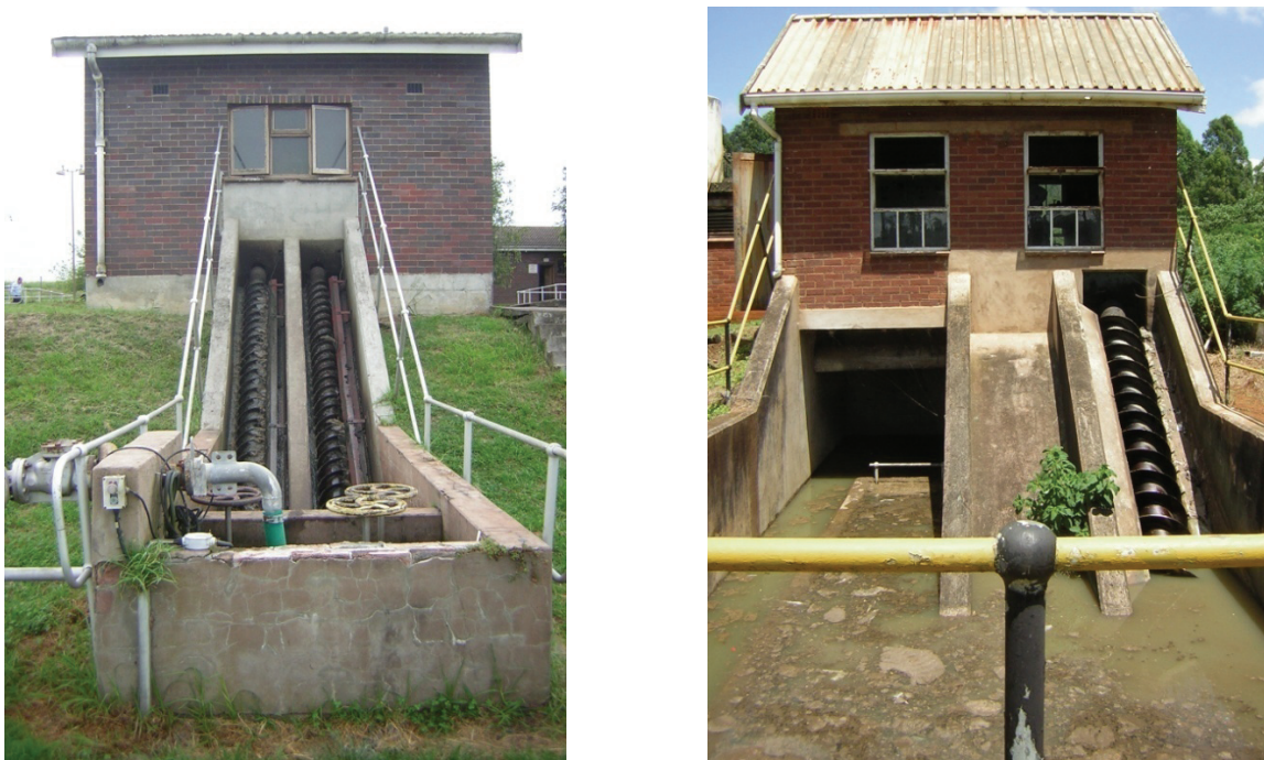
FIGURE 12.5.1: Typical Archimedian screw pumps
