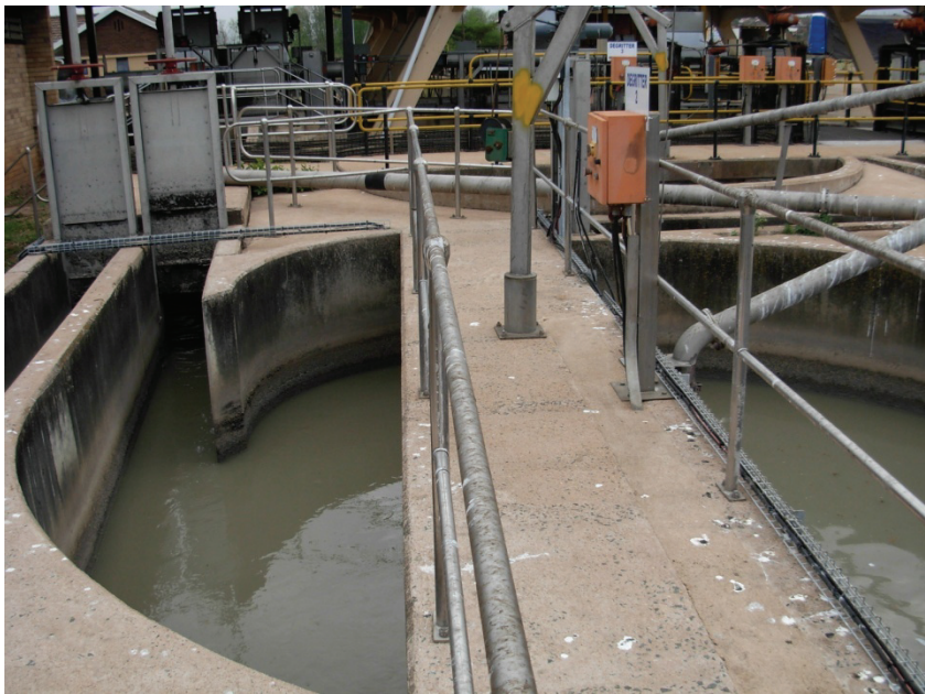
FIGURE 3.3.1: Typical vortex-type grit chamber
