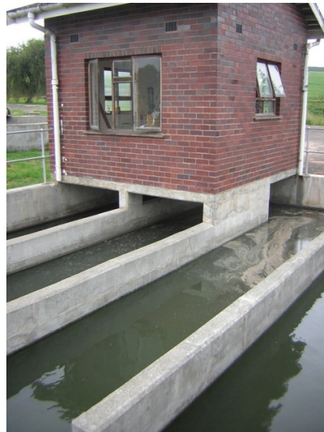
FIGURE 10.1: Typical chlorine contact tank
