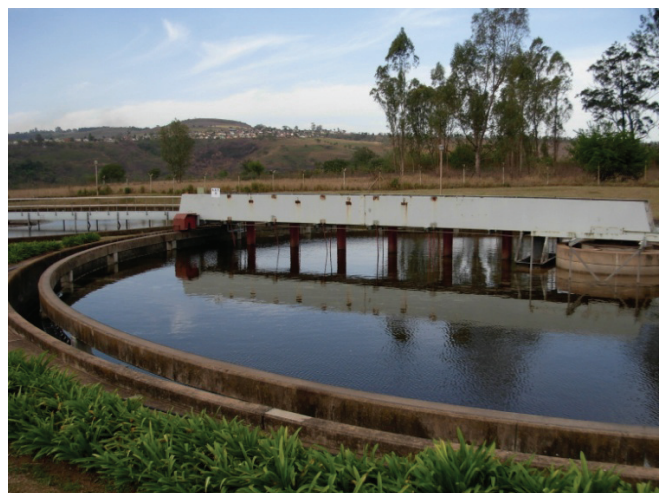
FIGURE 6.3.2: Typical secondary sedimentation tanks
