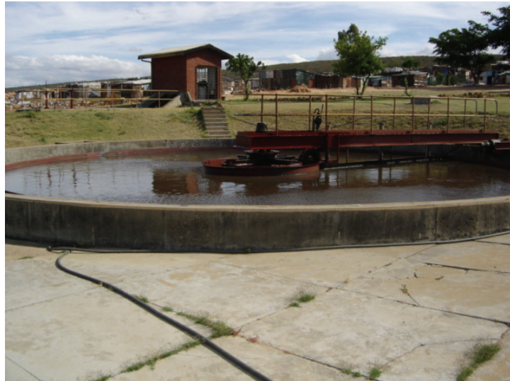
FIGURE 6.3.1: Typical primary settling tank (courtesy eWISA)
