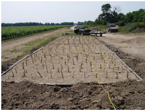
FIGURE 5.6.1: Artificial reedbed under construction
