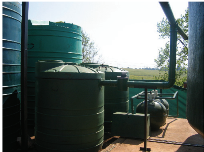
FIGURE 8.4.1: Typical submerged media reactor
