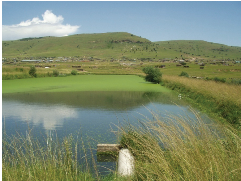
FIGURE 5.3.1: Typical maturation pond
