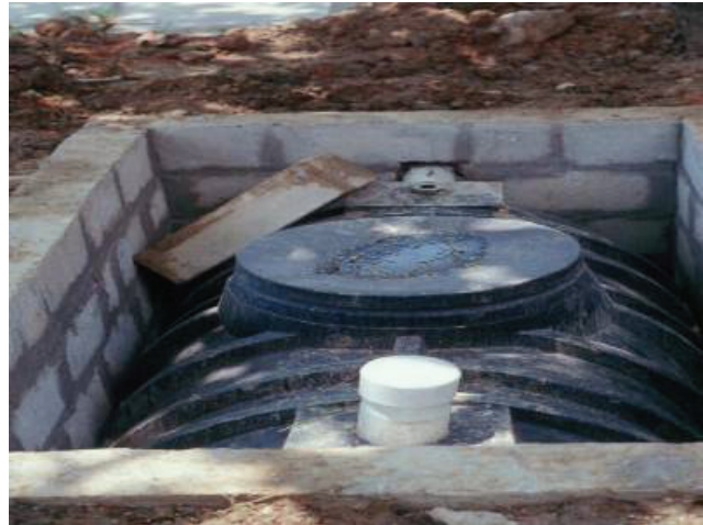
FIGURE 4.1.2: Partially installed septic tank
