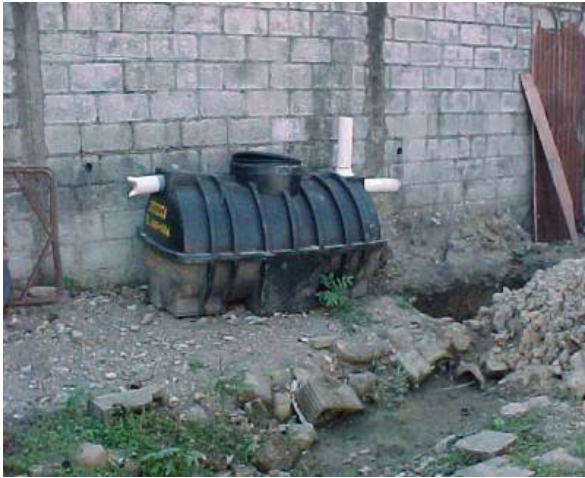
FIGURE 4.1.1: Septic tank before installation
