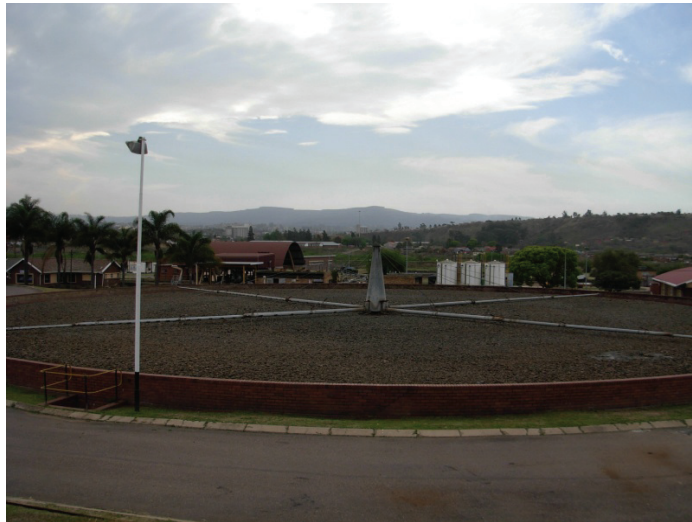
FIGURE 8.1.1: Typical trickling filter
