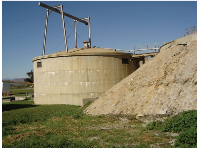
FIGURE 9.2.1: Typical anaerobic digester (eWISA)
