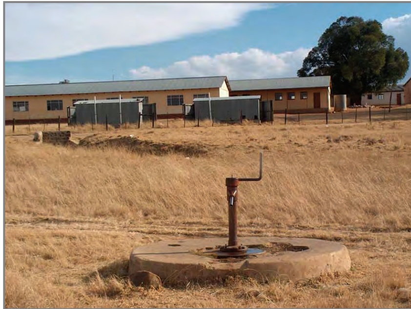
Plate 13: A poorly sited borehole near a school pit latrine (Photo by R Murray)
