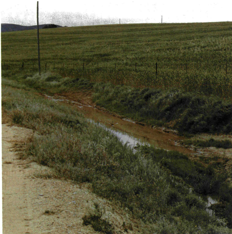
Surface flow being diverted from the dam.
